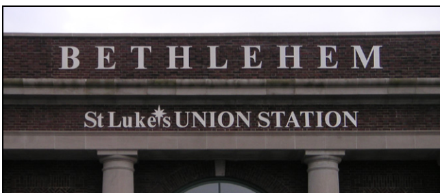
The letters have been individually pin-mounted to the parapet and frieze of the building. The color of the letters strongly contrasts the brick, making it clearly legible. The historic function of the building as a train station is also recognized in the name.
