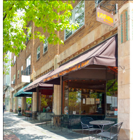
These closed-sided awnings are sized to fit between the masonry piers and provides shelter for pedestrians, advertisement for the businesses, and reduces the effect of the sun's rays at the interior.
