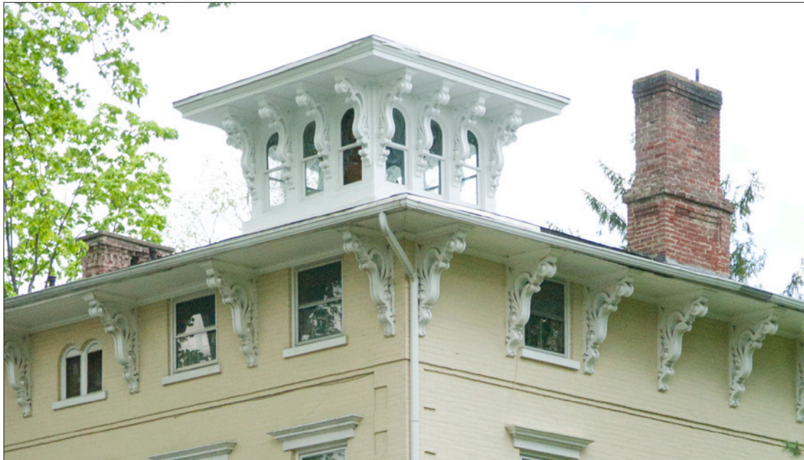
Roofs and roof-related features often frame the silhouette of a building against the sky and can help to define a building's style. This Italianate house includes a distinctive central cupola with three half-round headed windows at each face and a projecting, bracketed cornice. The flanking brick chimneys include recessed "paneled" bases. The brackets at the projecting main cornice frame third floor window openings.
