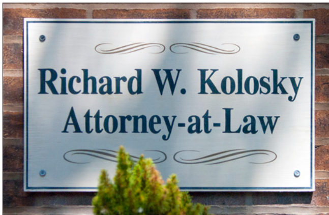
This small-scale, professional services sign includes a clear message, serif-style lettering and a pin stripe border, providing a finished appearance. The screws are fastened into mortar joints.
