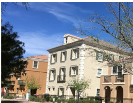
New Construction 4-Story Condo Building
