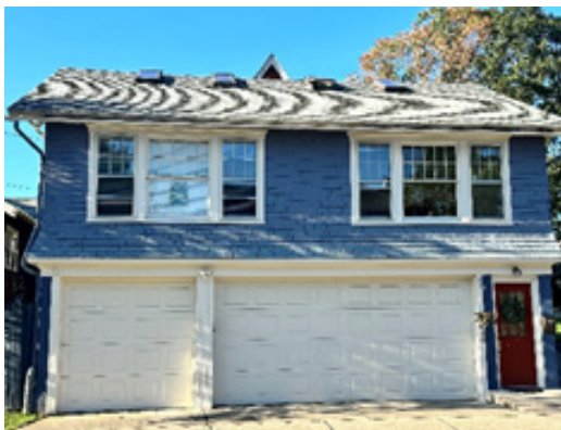
Garage Apartment in Bethlehem, PA
