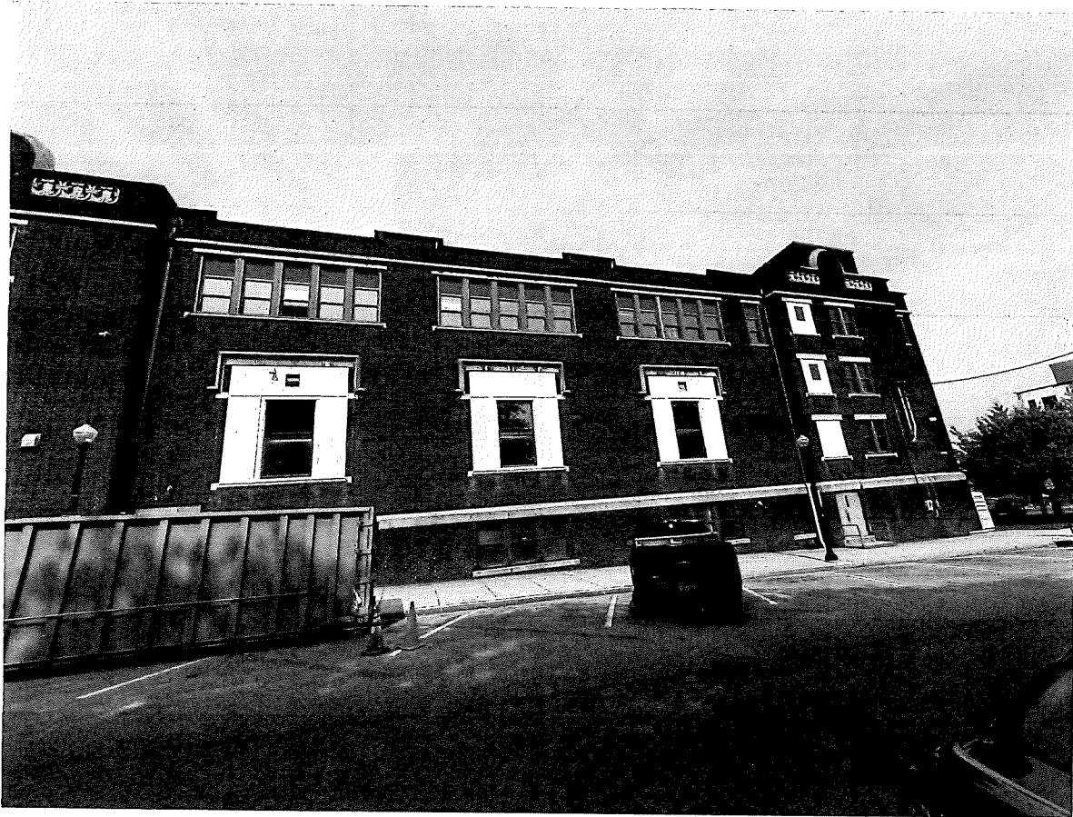
Exterior Webster Street
