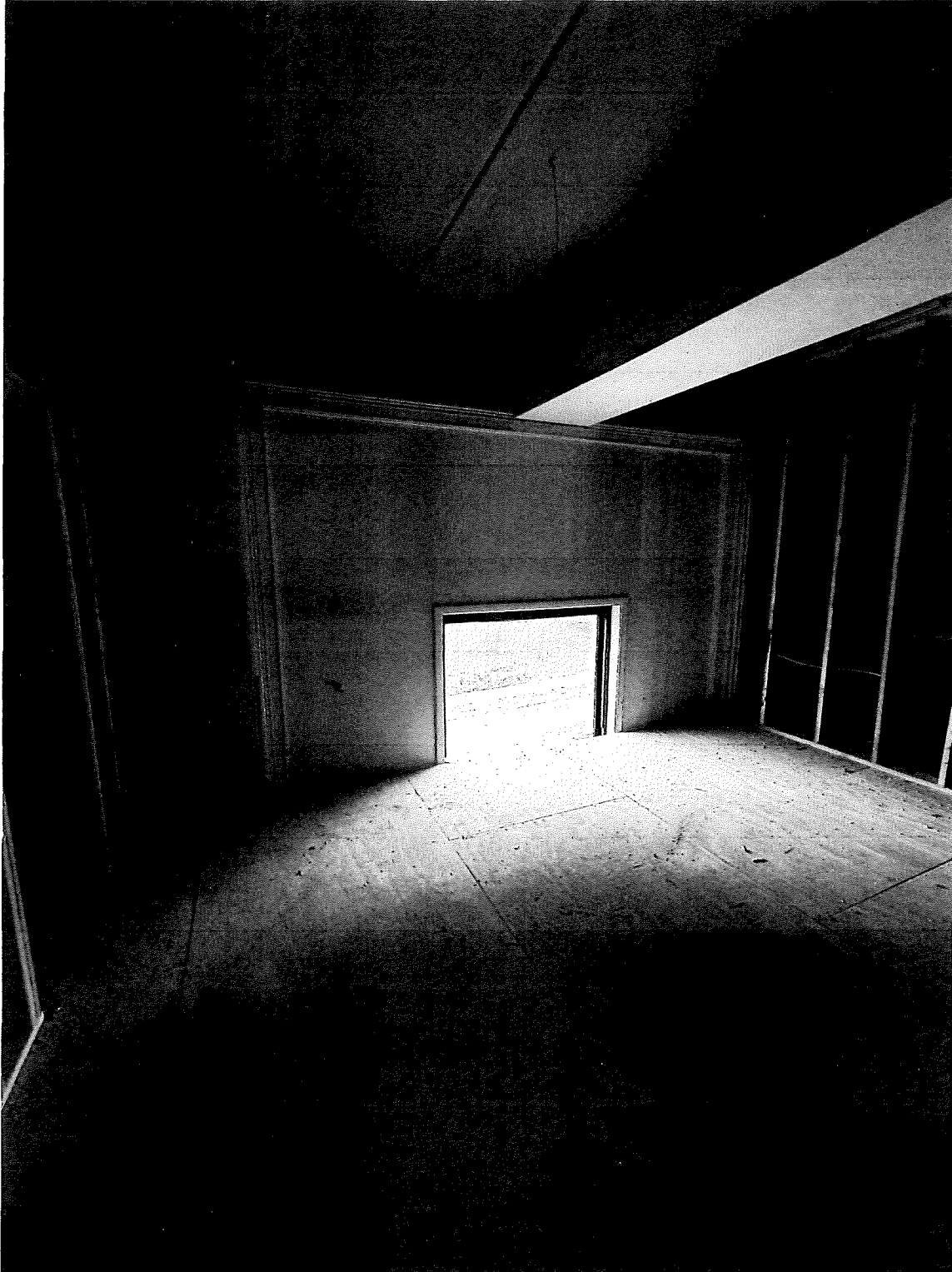
Third Floor Existing Interior
