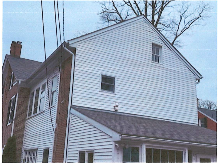
Area outlined in red to be restored. There is original brick underneath the vinyl siding.
