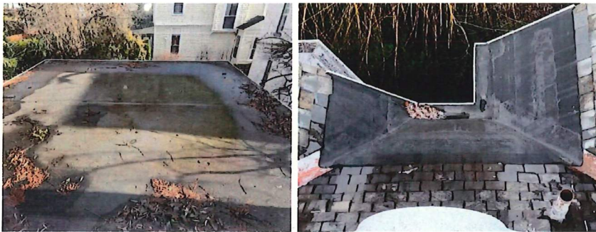
Built-up Roof: Built up roof with gravel
