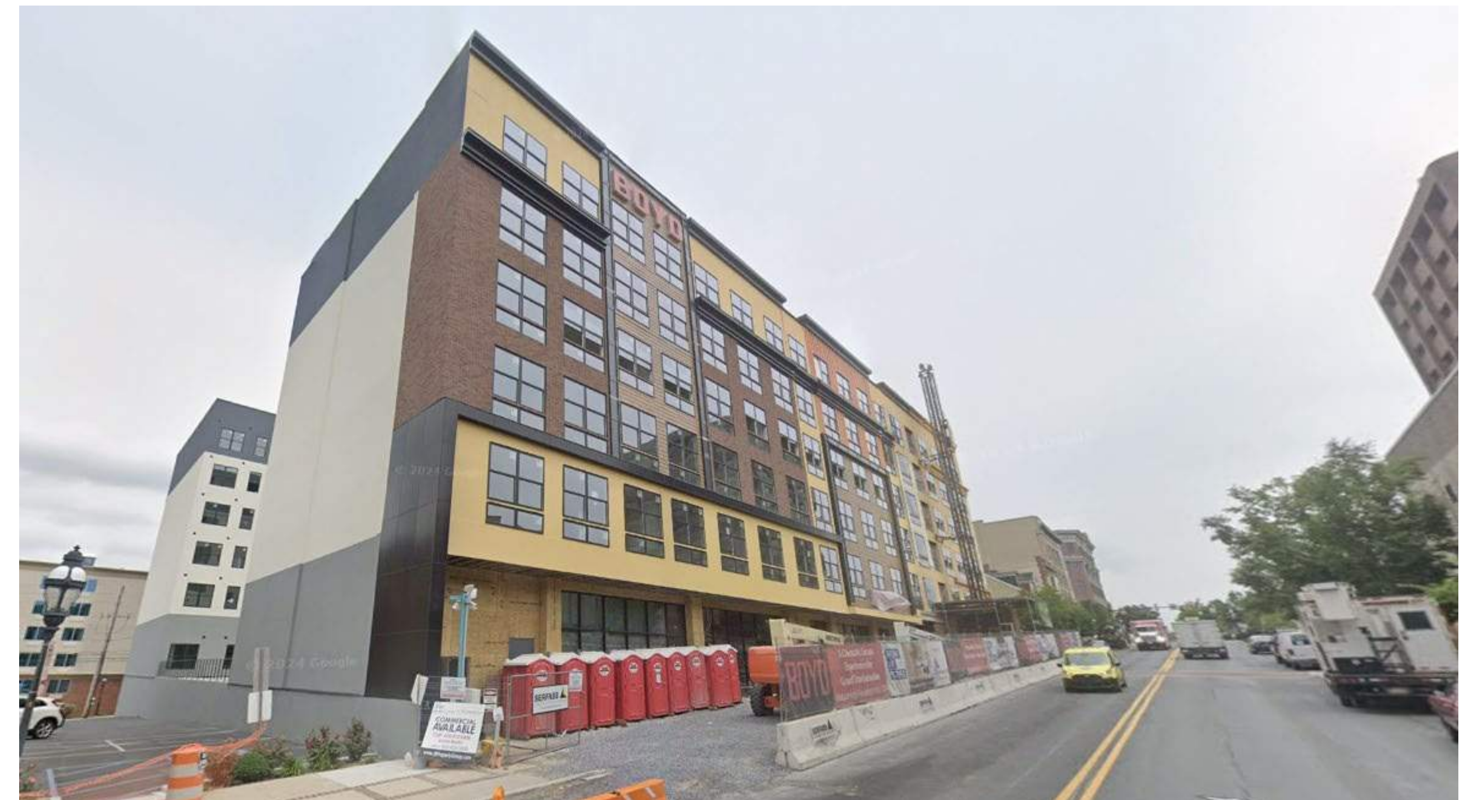
VIEW LOOKING EAST FROM W BROAD STREET - BOYD APARTMENT BUILDING
