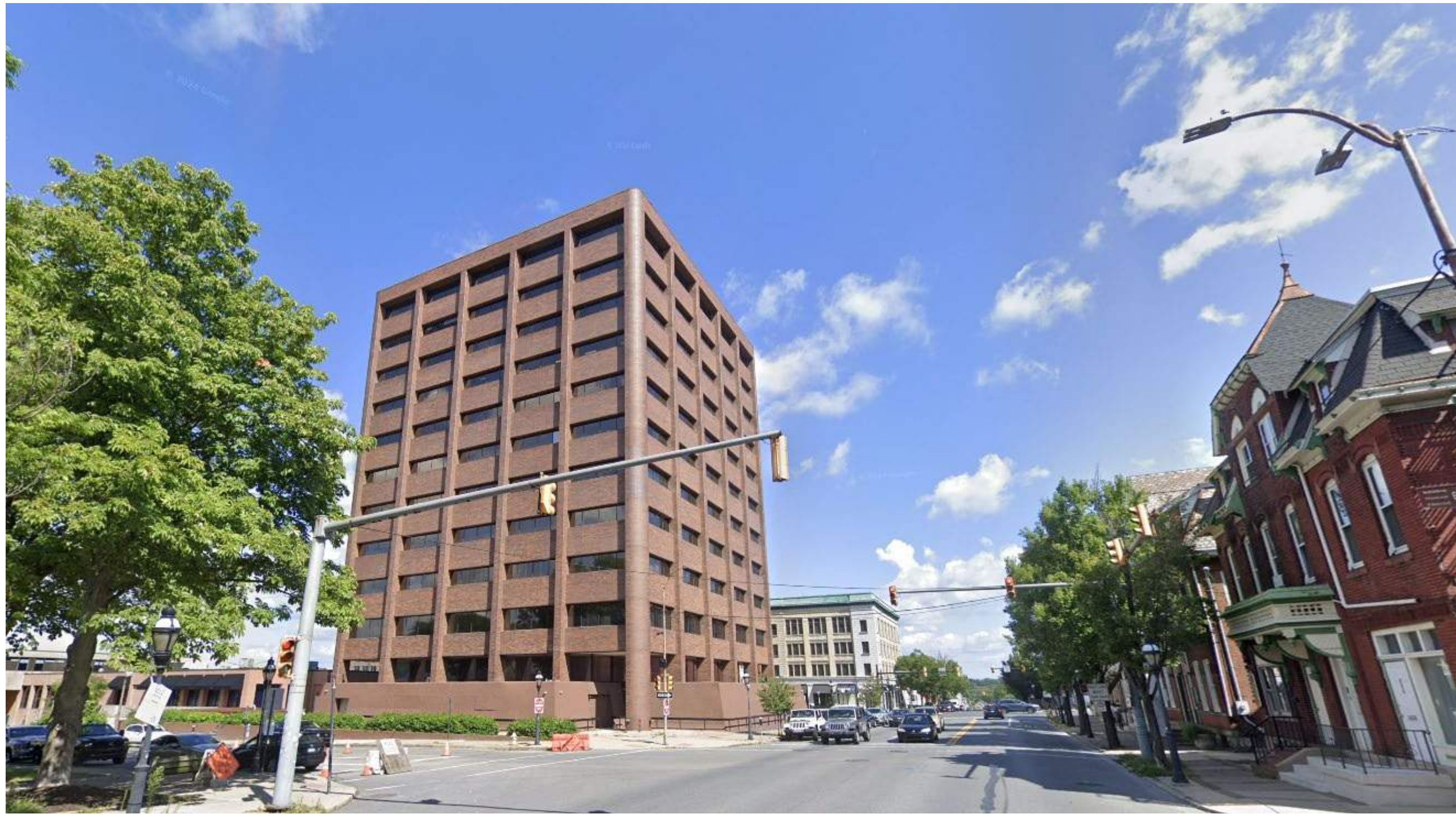
VIEW LOOKING NORTH FROM N NEW ST & W WALNUT ST - ONE BETHLEHEM PLAZA
