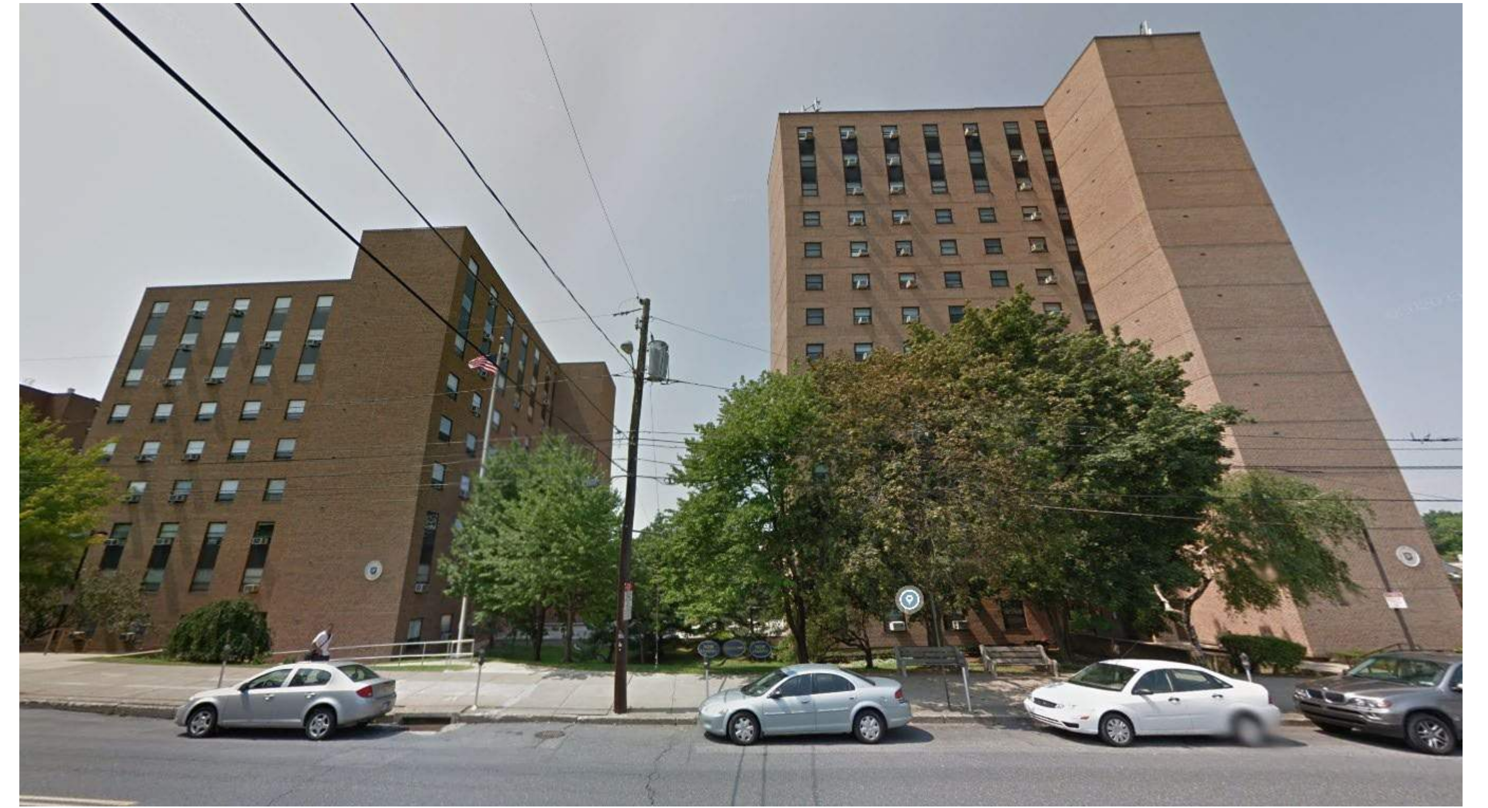
VIEW LOOKING WEST FROM MAIN ST. & W GARRISON ST - MORAVIAN HOUSE & OLD YORK CENTER
