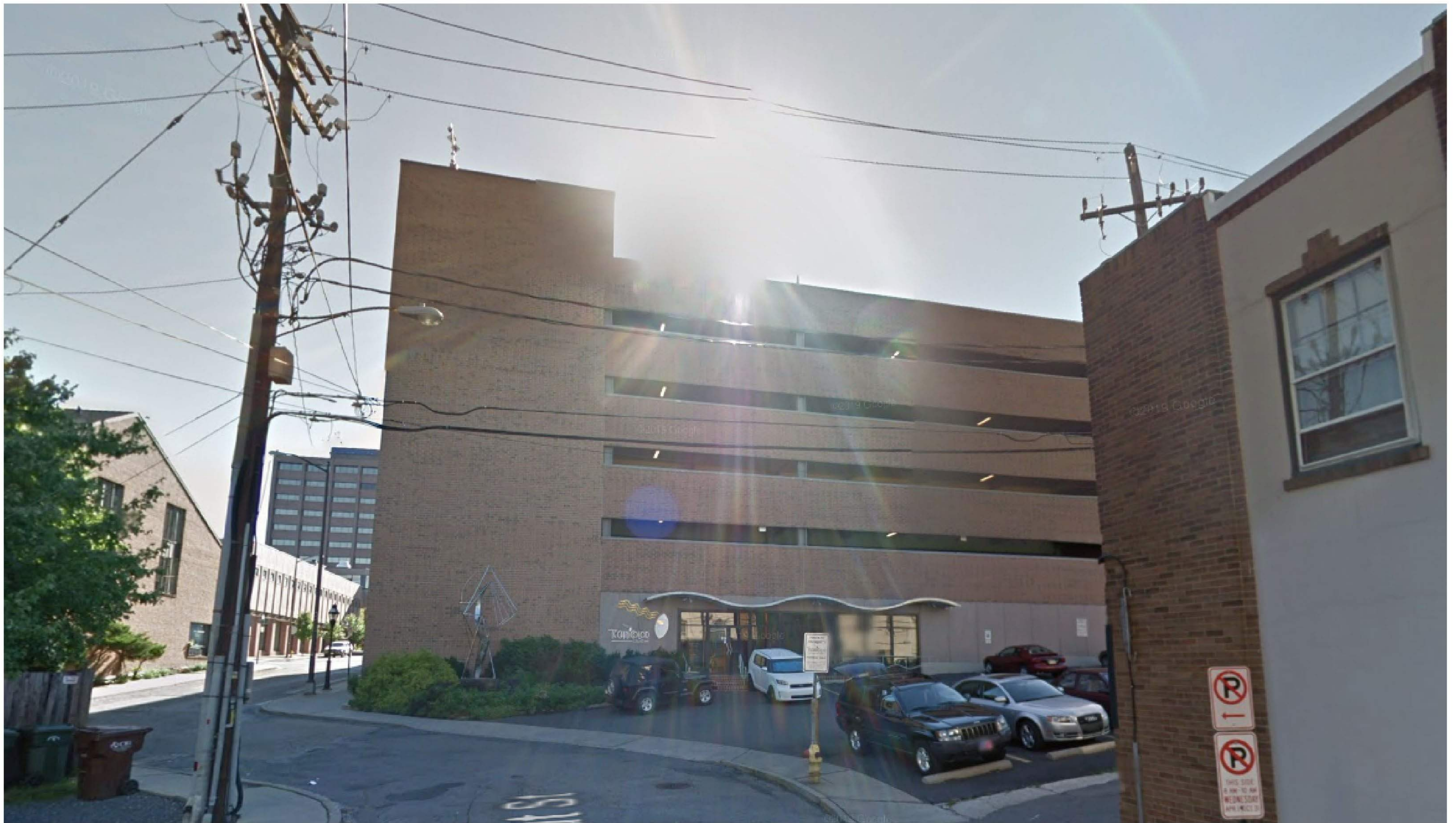
EXISTING VIEW LOOKING EAST FROM W WALNUT STREET
