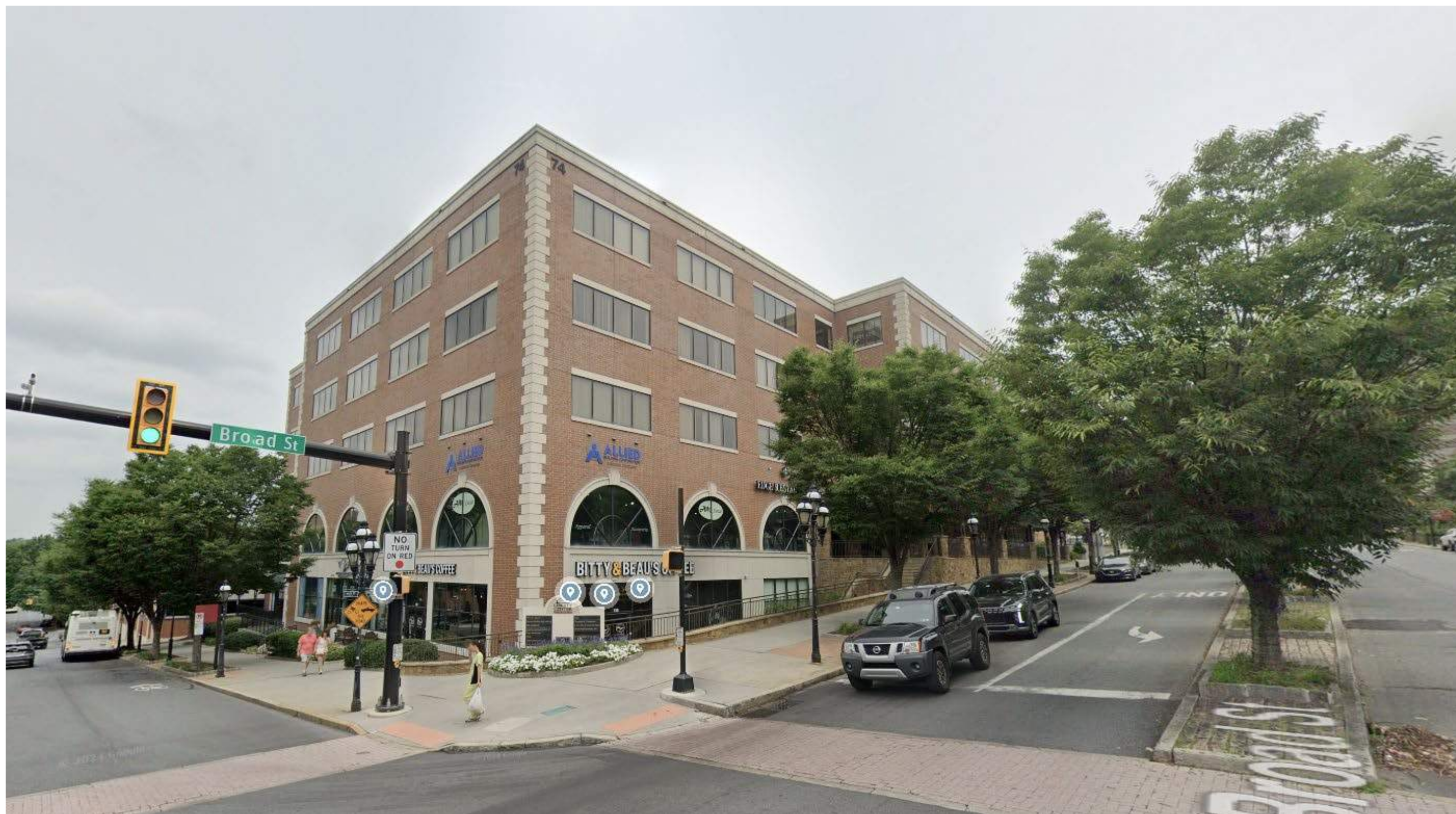
VIEW LOOKING EAST W BROAD STREET - 74 W BROAD STREET
