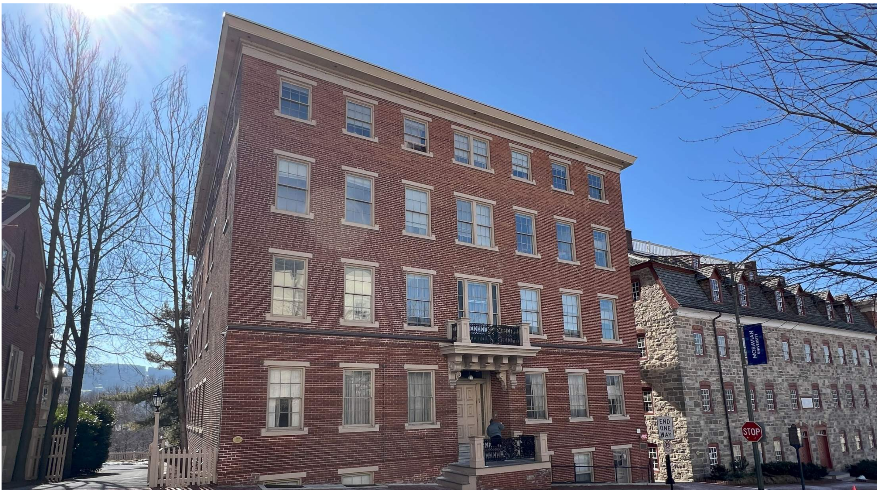
VIEW LOOKING EAST FROM W CHURCH ST AND MAIN ST - 85 W CHURCH ST
