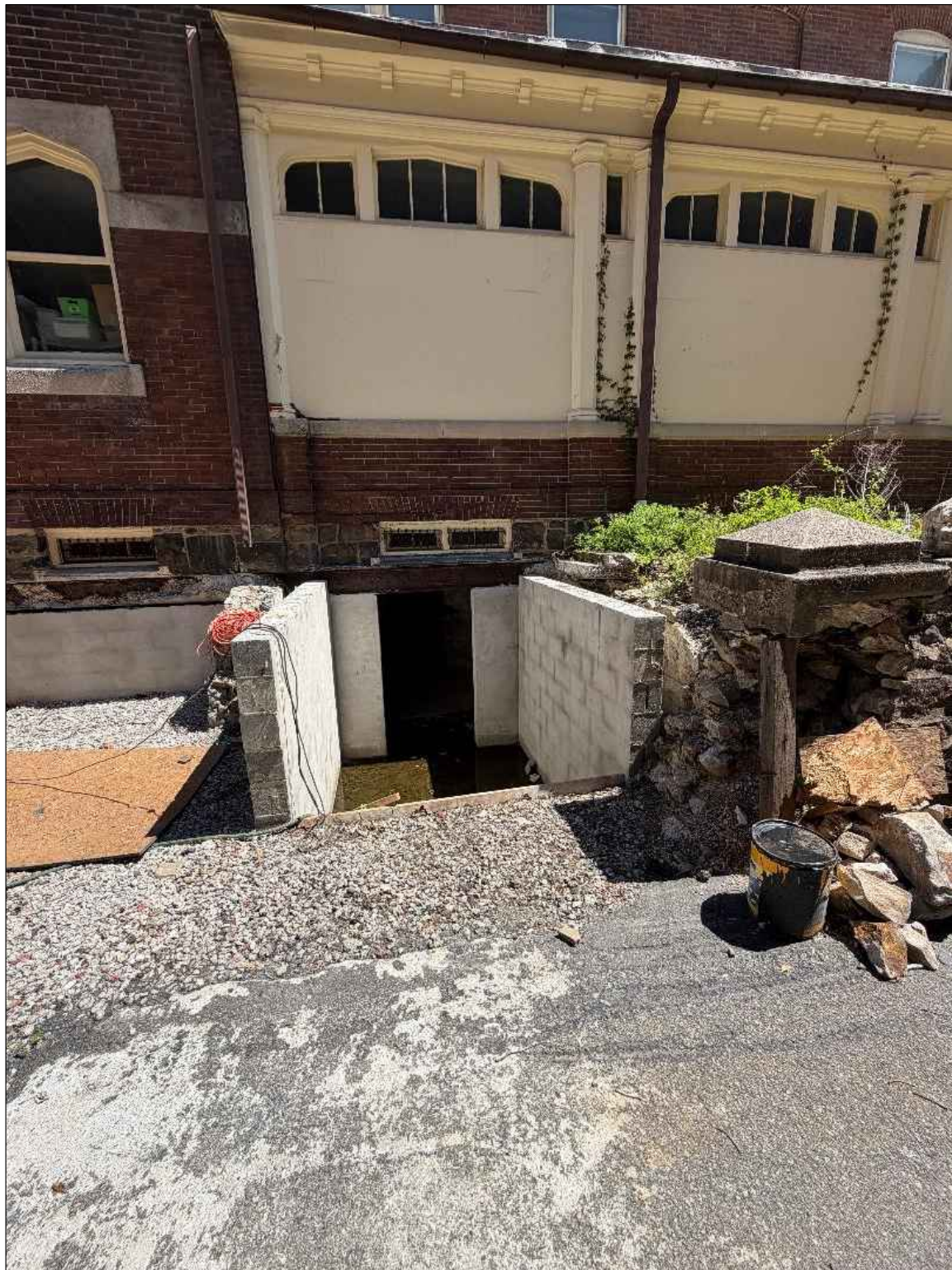
CURRENT CONDITION LOOKING TOWARD EXISTING BASEMENT OPENING
