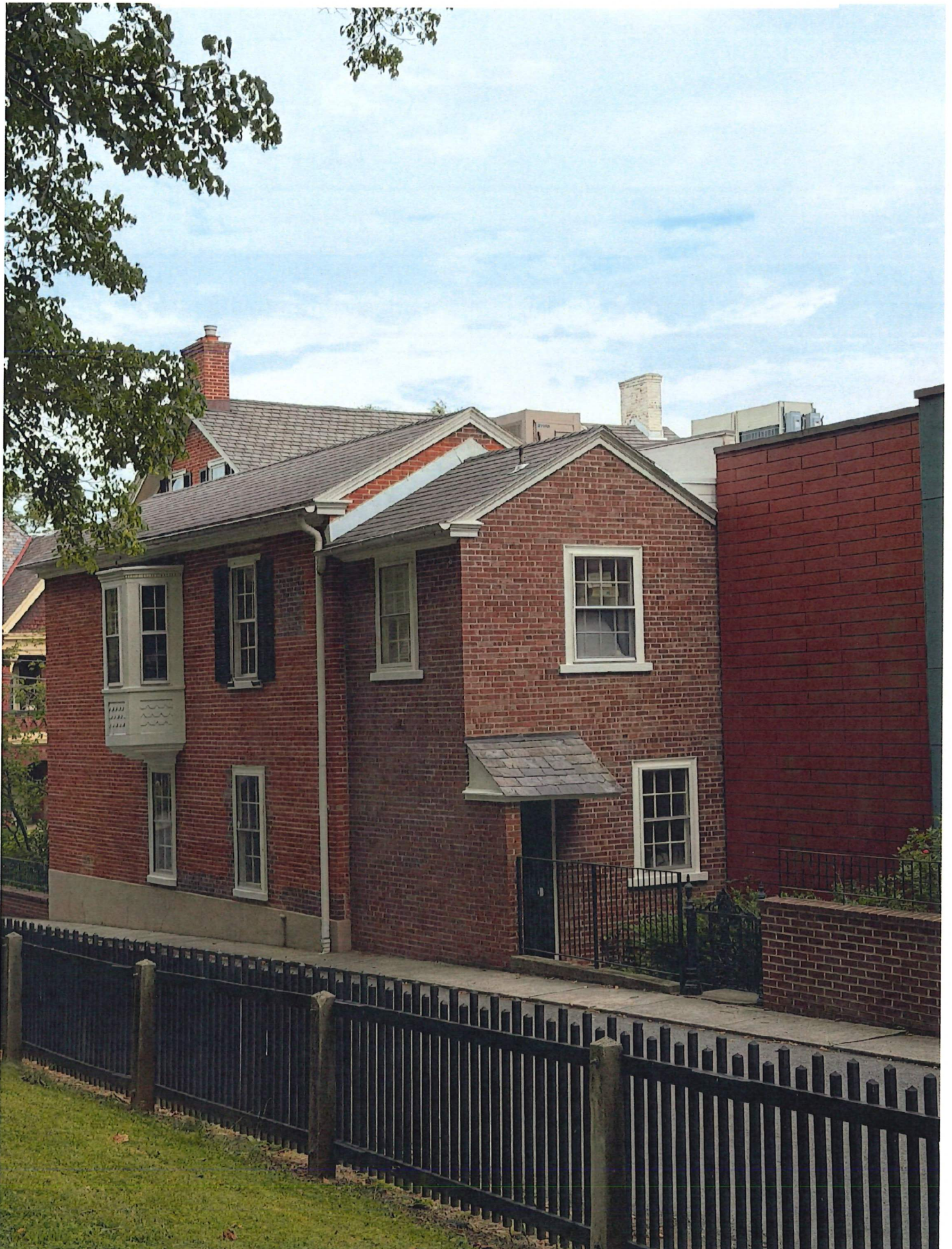
Northside section – “Slateline” shingles
