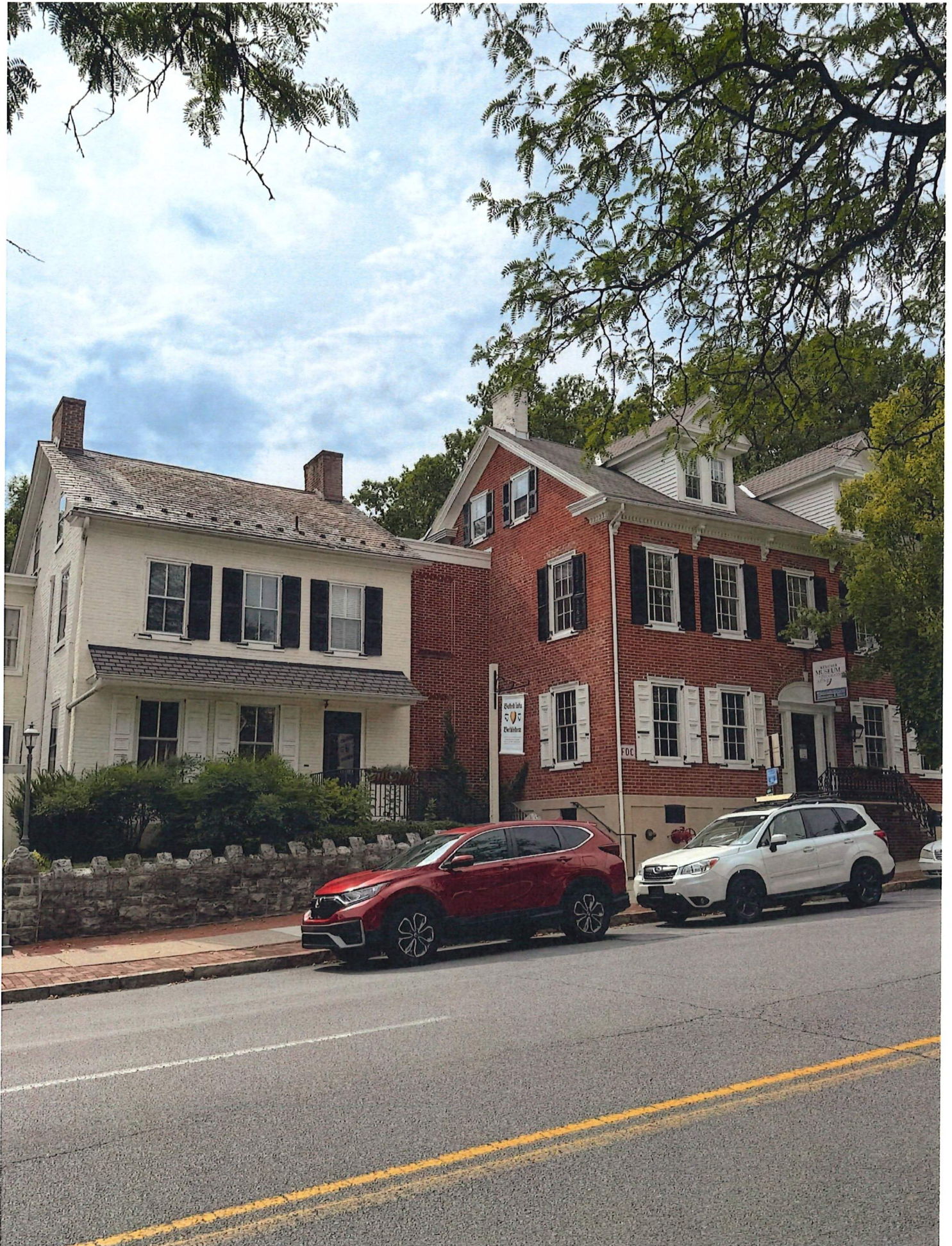
Slate Roof on left, "Slateline" on right roof and on Pent roof
