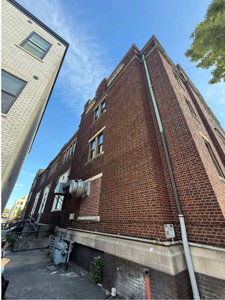
WEST FACADE - before the ada ramp.
