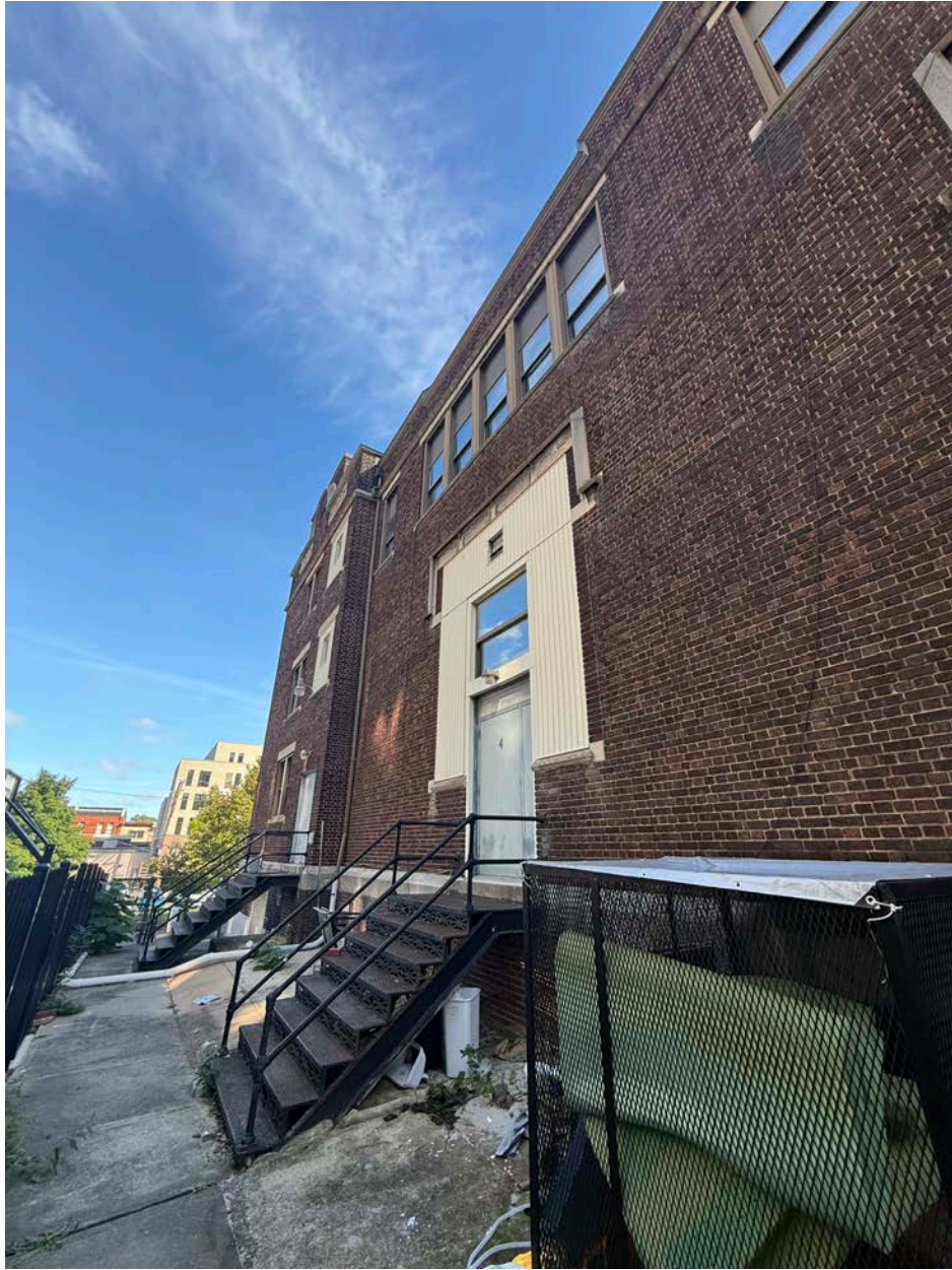
WEST FACADE - after ada ramp.
