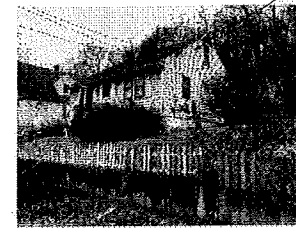
Existing Conditions Photo Not To Scale
