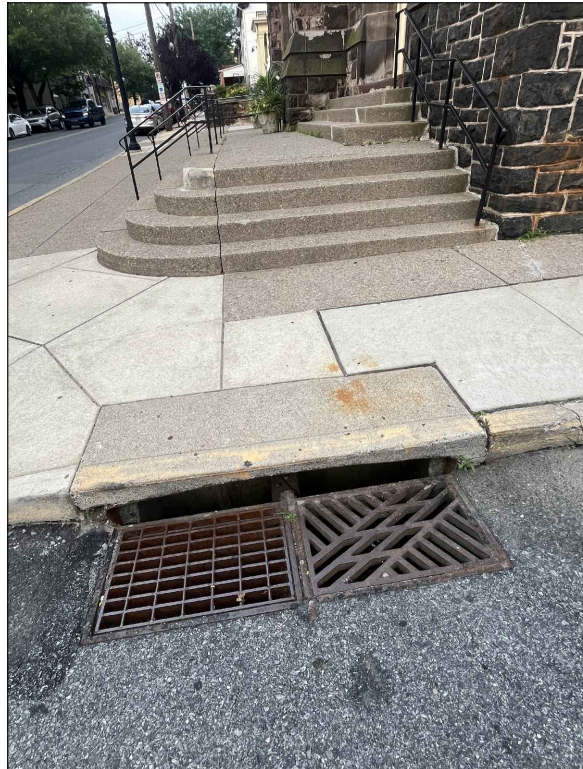
WEST ELEVATION LOOKING EAST
