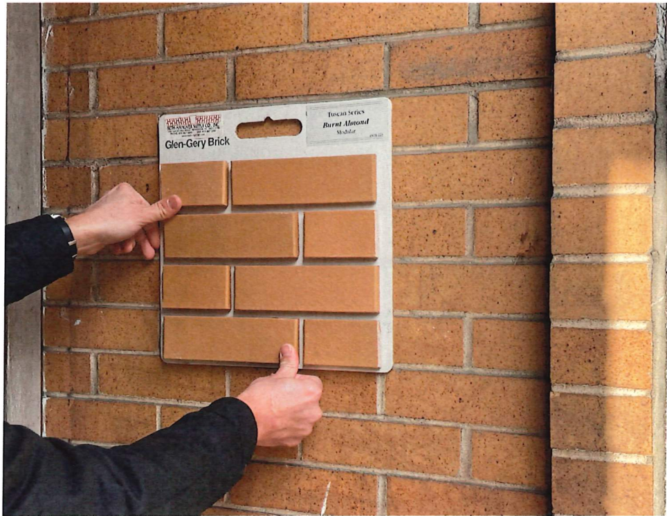
GLEN-GERY BRICK (TUSCAN SERIES: BURNT ALMOND MODULAR) AT GROUND LEVEL
