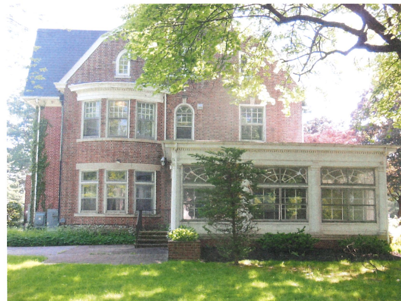
C WEST FACADE - 12TH AVENUE
