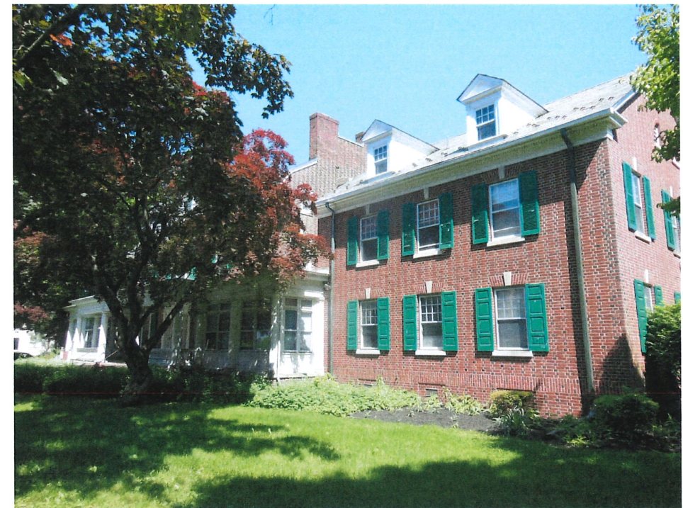
B SOUTHEAST FACADE - PROSPECT AVENUE
