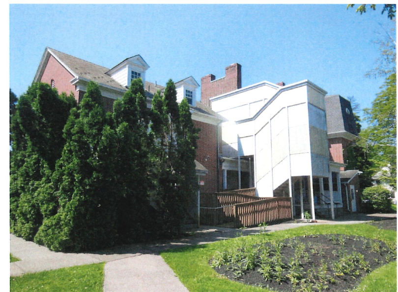
F NORTHEAST FACADE - W. MARKET STREET
