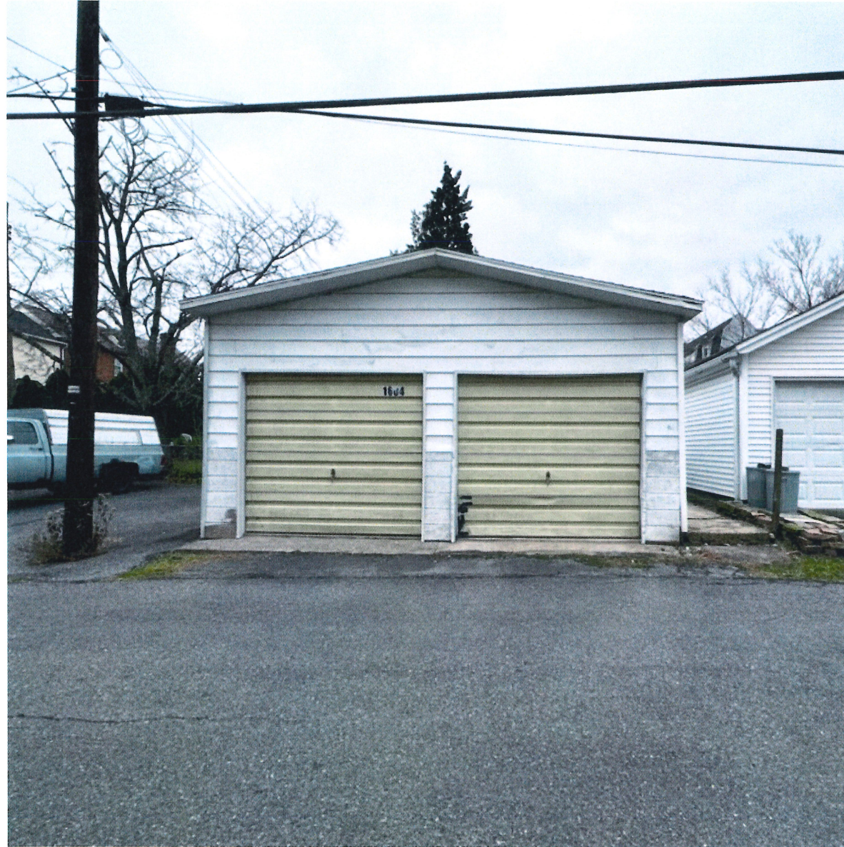
3. Garage to be demolished
