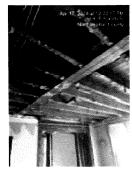
Exposed Joists in Ceiling of "Dining Room" – note also Steel Bearing Beam
