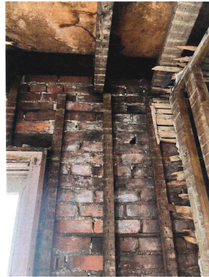
Typical Exposed Brickwork
