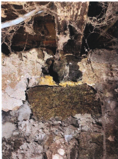
Joist Support on Foundation Wall
