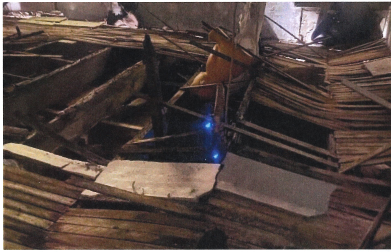
Interior of Garage
