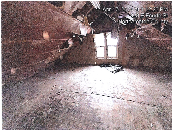
3rd Floor Attic
