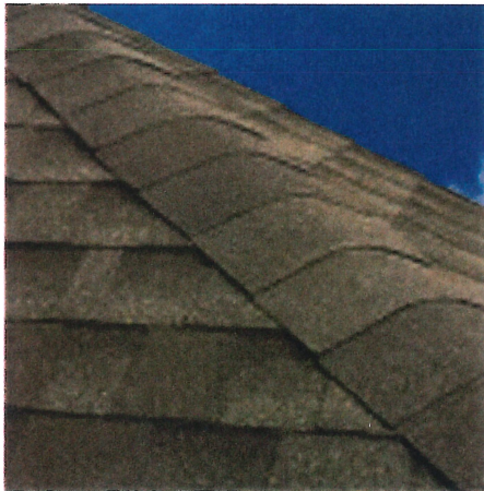
Before Cut-up 3-tab strip shingles used at the hips and ridges.
