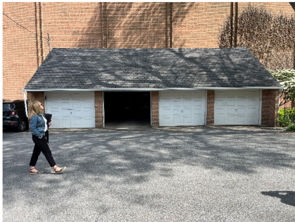
South façade of residential 4-car garage
