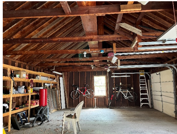
Interior; wood framing
