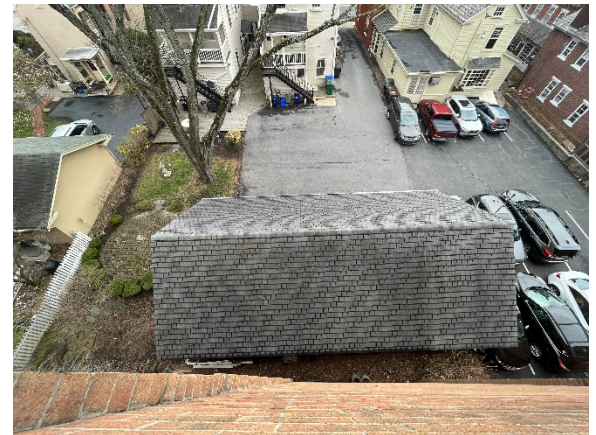
Shingle roof; close proximity
