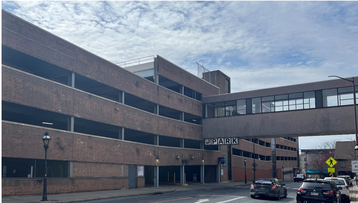
North Elevation / Walnut Street Façade
