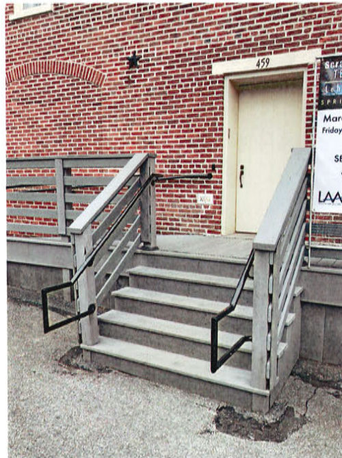
g. North Elevation, detail of existing egress steps
