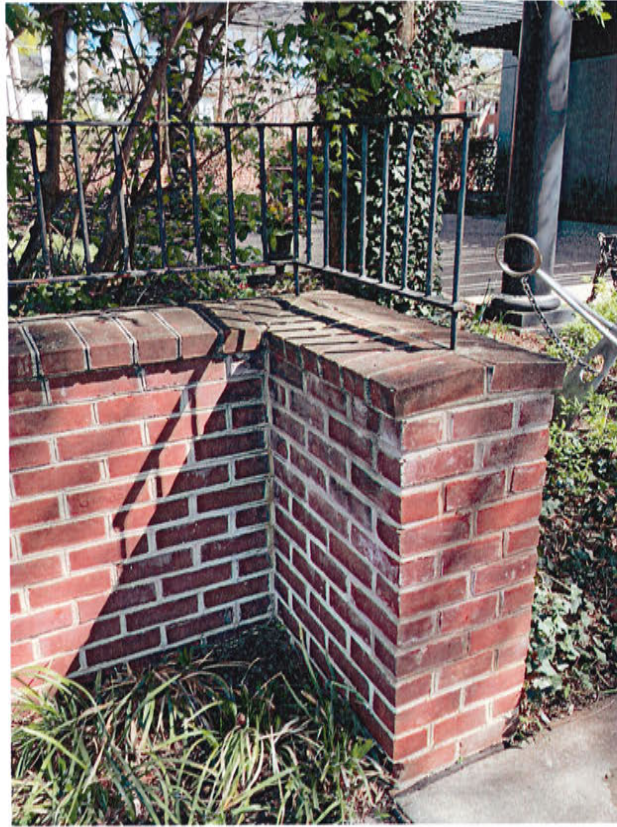
h. Existing (brick) garden wall at rear property perimeter, corner detail
