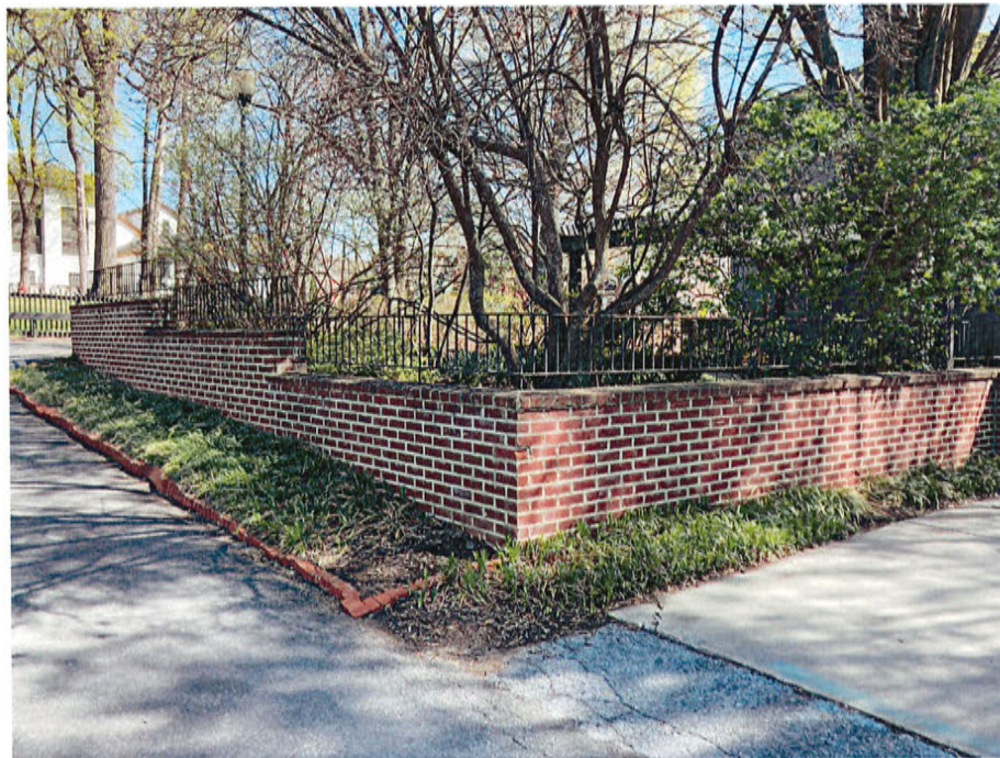
g. Existing (brick) garden wall at rear property perimeter
