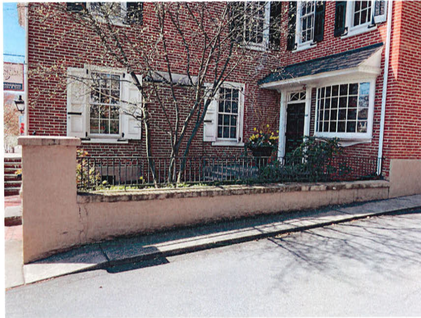
f. Existing (block) garden wall at North Elevation (northeast corner)
