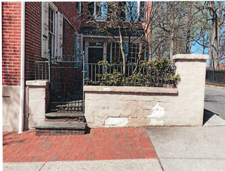
e. Existing (block) garden wall at East Elevation (northeast corner)
