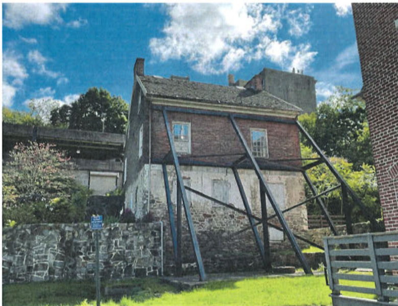
West Façade of House; Steel Shoring visible (c. 2007) – one column at right will remain to be used to support the Overlook Gallery (the rest of the steel structure will be removed once the House is structurally reinforced in Phase 1)
