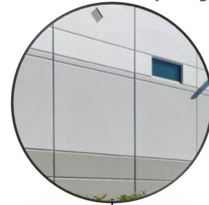
STAIN PRECAST CONCRETE (to make artificial openings)
