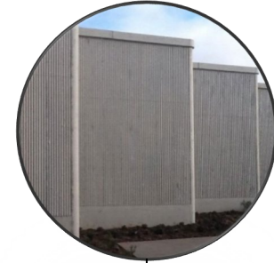
PRECAST WITH FORM LINERS
