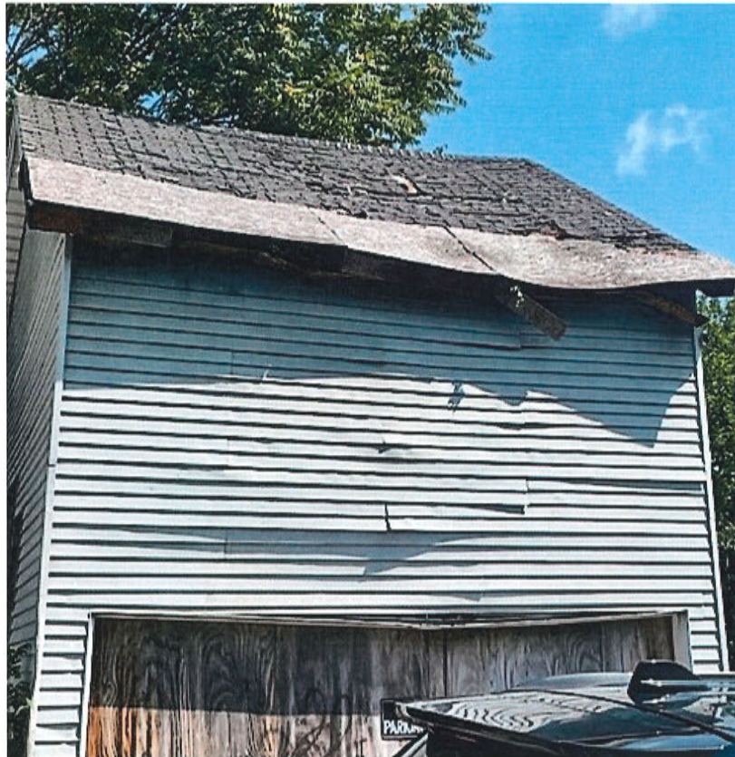
Figure 6: Existing Condition – Unstable Roof
