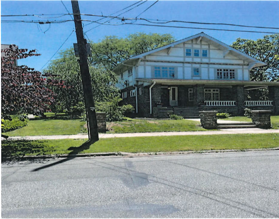
From Top: driveway, across the street, right side, backyard, front and front/left corner
