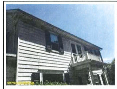
Install gutters on both sides of front porch roof.
