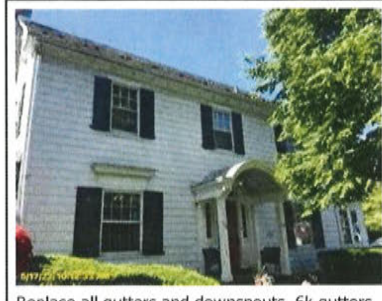
Replace all gutters and downspouts. 6k gutters with 3x4 downspouts in black.
