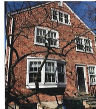
View of south side
