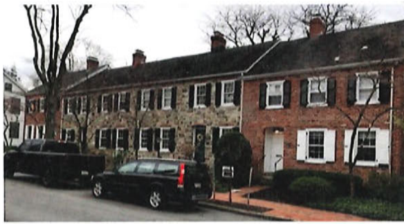
View from Wall Street of 58, 56, 54, and 52 E. Wall St. (at right)
