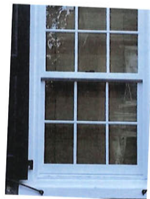
View from Wall St of 54 E. Wall St with proposed Andersen 400 series window installed
