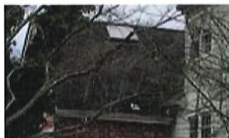
View of skylight on south-facing roof (top) and east-facing roof (bottom) of 52 E. Wall St
