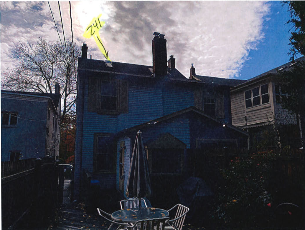
ALAN KUNSMAN ROOFING / TRAVIS / 01-12-22
