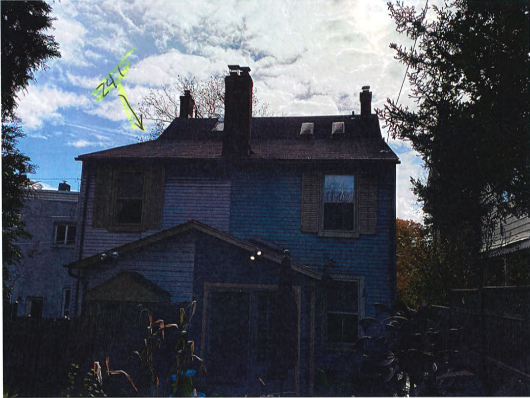
ALAN KUNSMAN ROOFING / TRAVIS / 01-12-22
