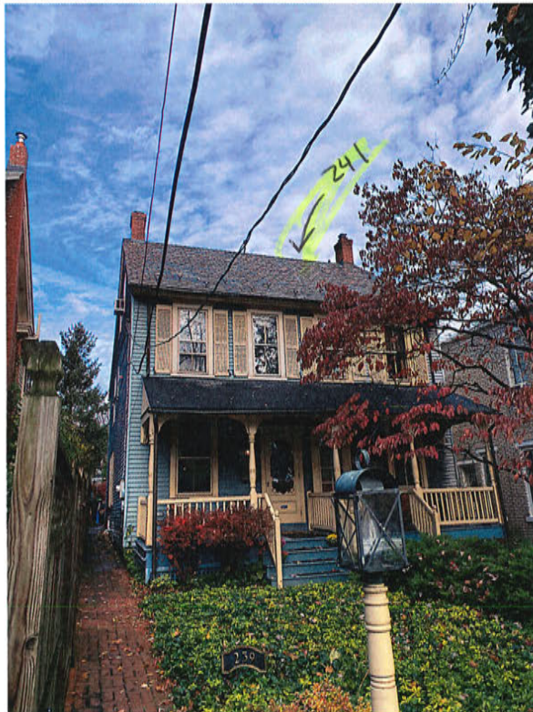
ALAN KUNSMAN ROOFING / TRAVIS / 01-12-22
