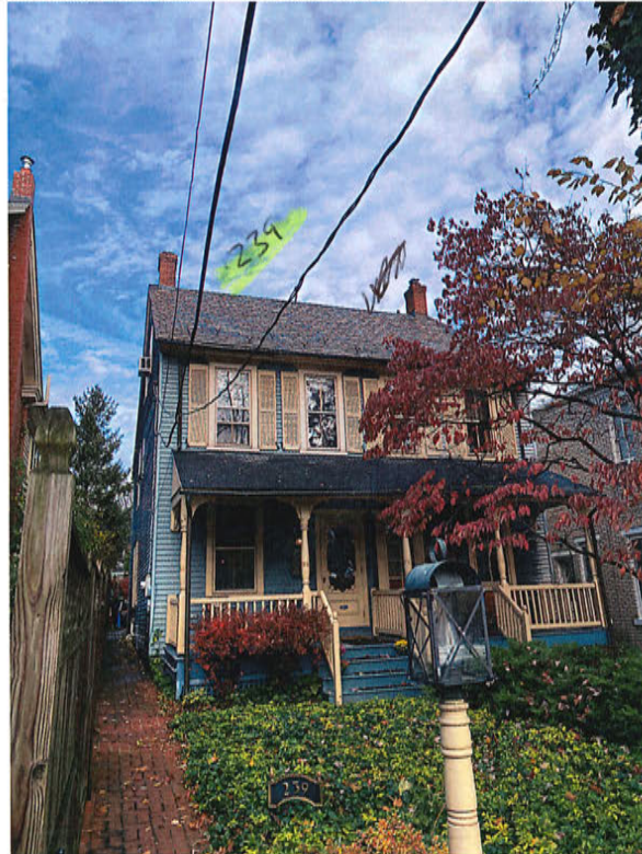
ALAN KUNSMAN ROOFING / TRAVIS / 01-12-22
