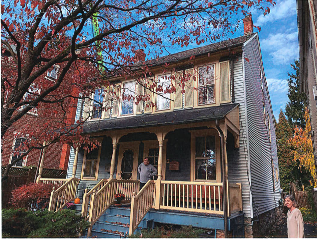
ALAN KUNSMAN ROOFING / TRAVIS / 01-12-22
