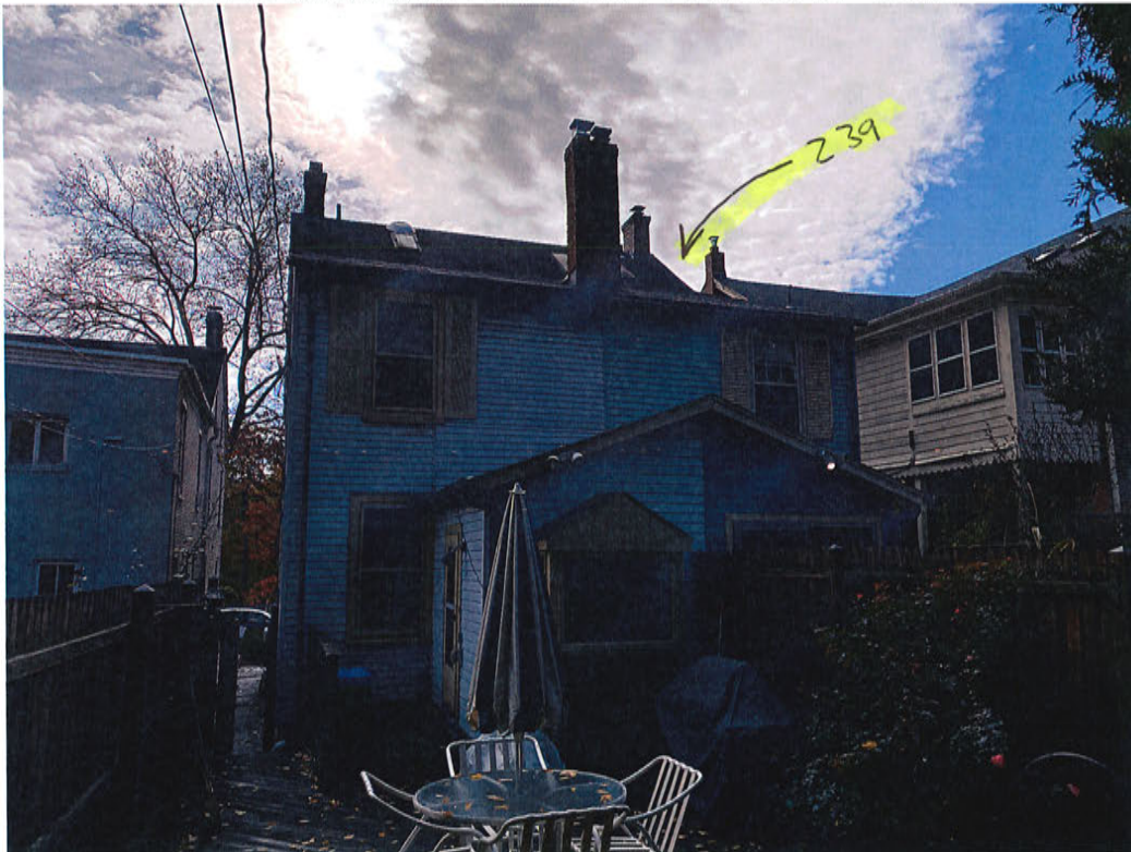
ALAN KUNSMAN ROOFING / TRAVIS / 01-12-22
