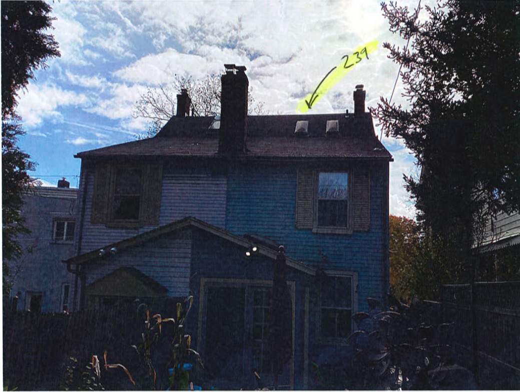
ALAN KUNSMAN ROOFING / TRAVIS / 01-12-22
