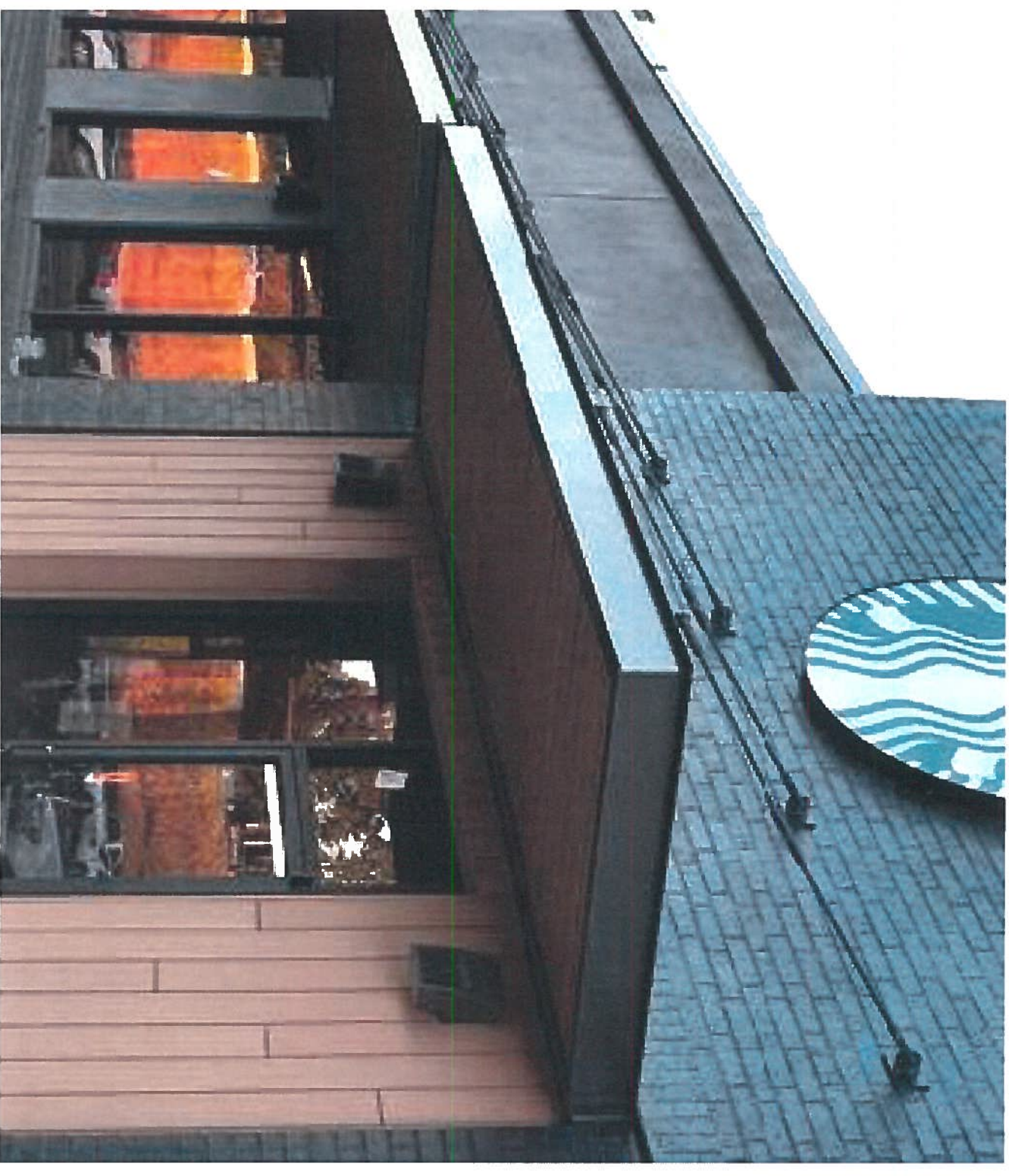
▶ SUSPENDED STEEL CANOPY AND "WOOD-LOOK" SOFFIT EXAMPLE
