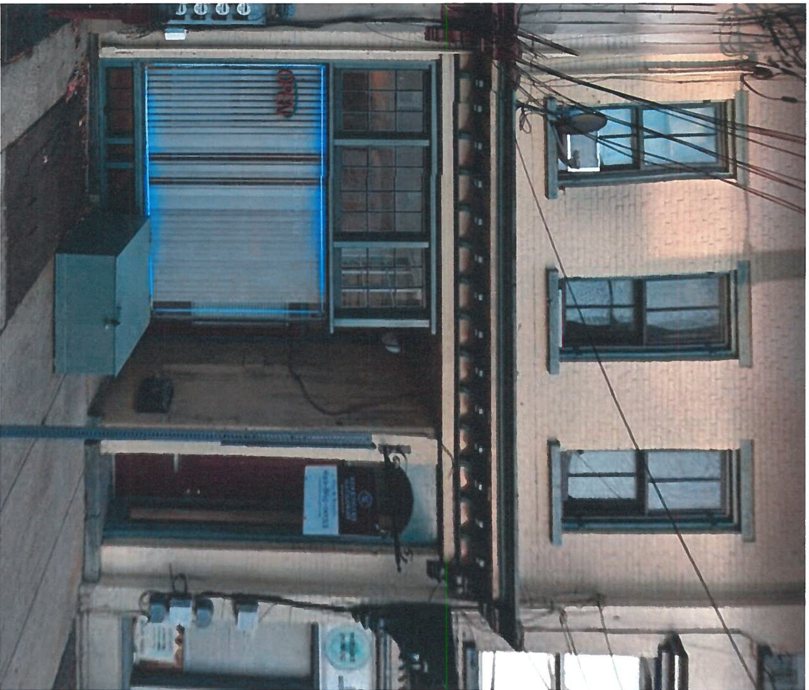
▶ SUSPENDED STEEL CANOPY AND "WOOD-LOOK" SOFFIT EXAMPLE
