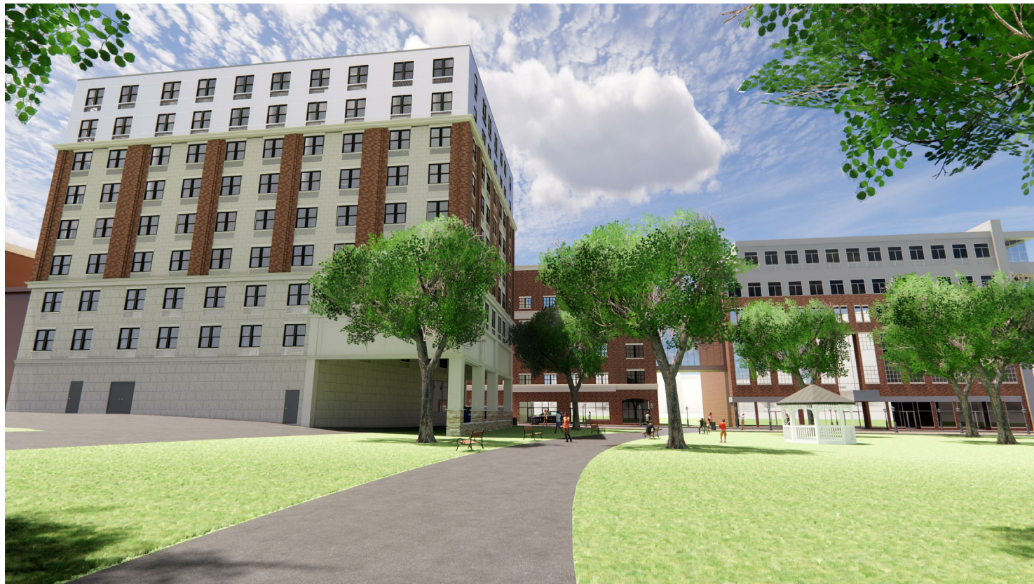
STREET VIEW LOOKING WEST FROM GREENWAY
