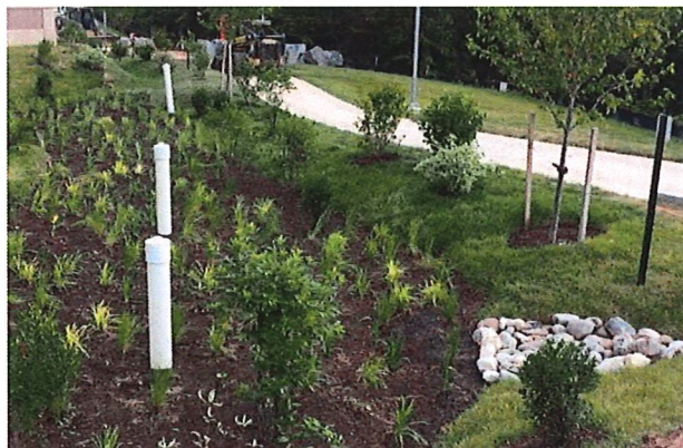
A stormwater structure, such as the bioretention facility above, may qualify a property owner for a credit on the stormwater utility fee.
