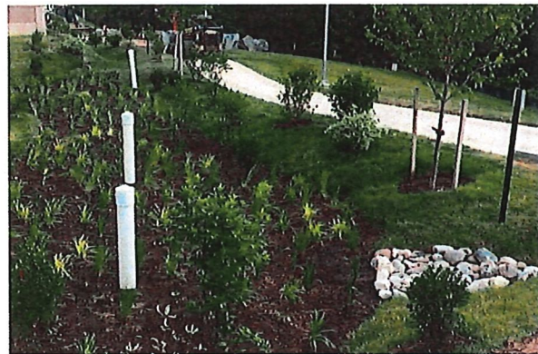
A stormwater structure, such as the bioretention facility above, may qualify a property owner for a credit on the stormwater utility fee.
