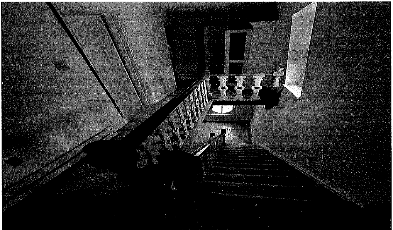
Standing at top of steps on third floor. 2 doors on the right are closet/storage. The back door on left leads into bedroom #1. The first door on the left leads into bedroom #3.
