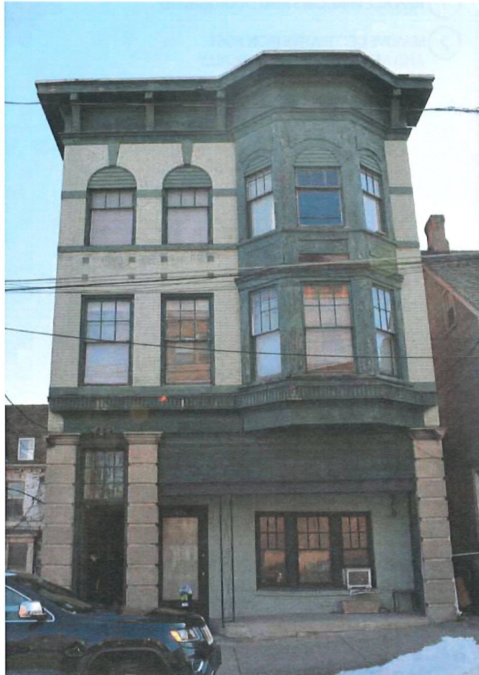
View of Existing Primary (East) Facade, Looking West
