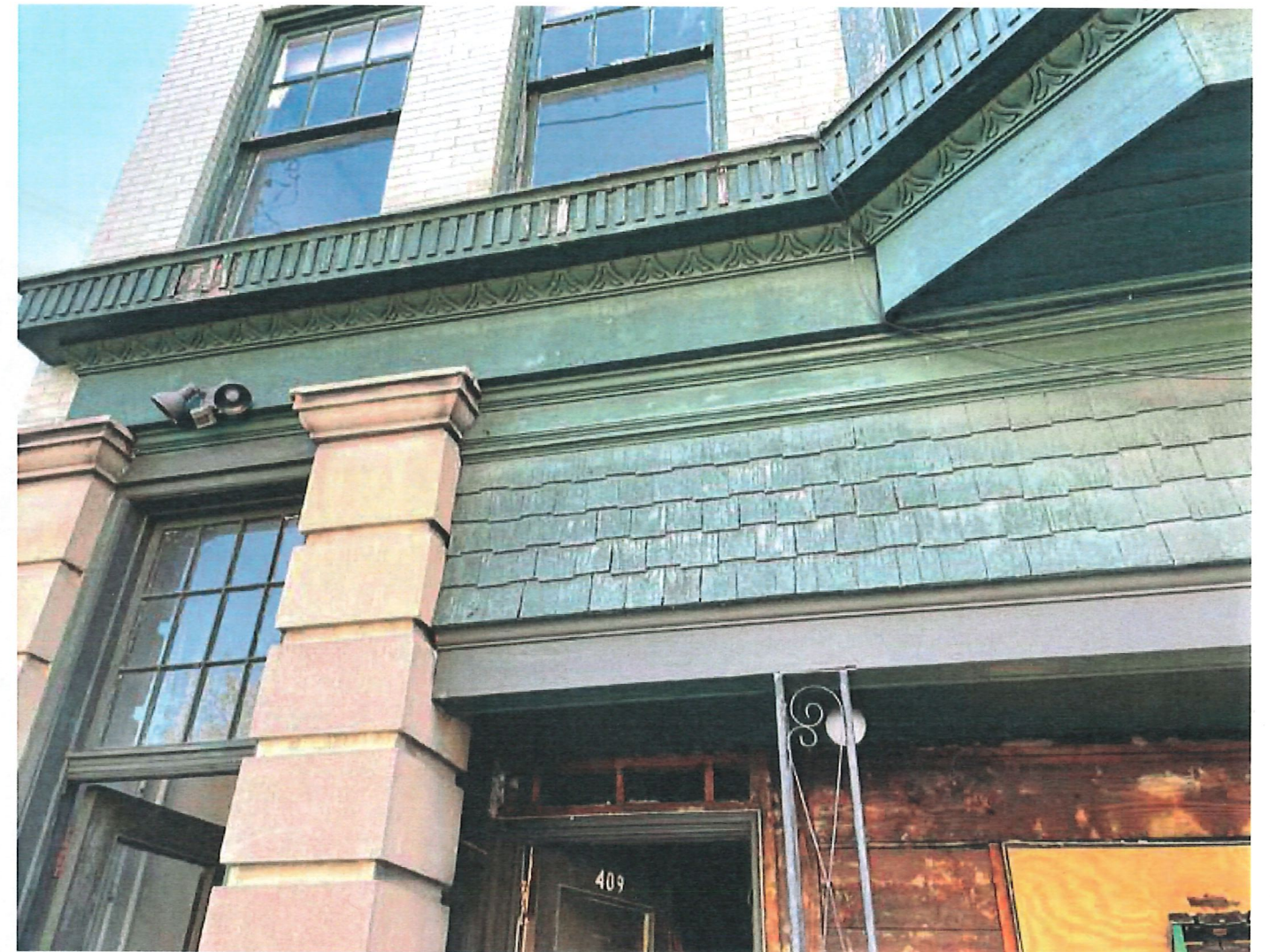
Close-up View of Transom Existing Siding
