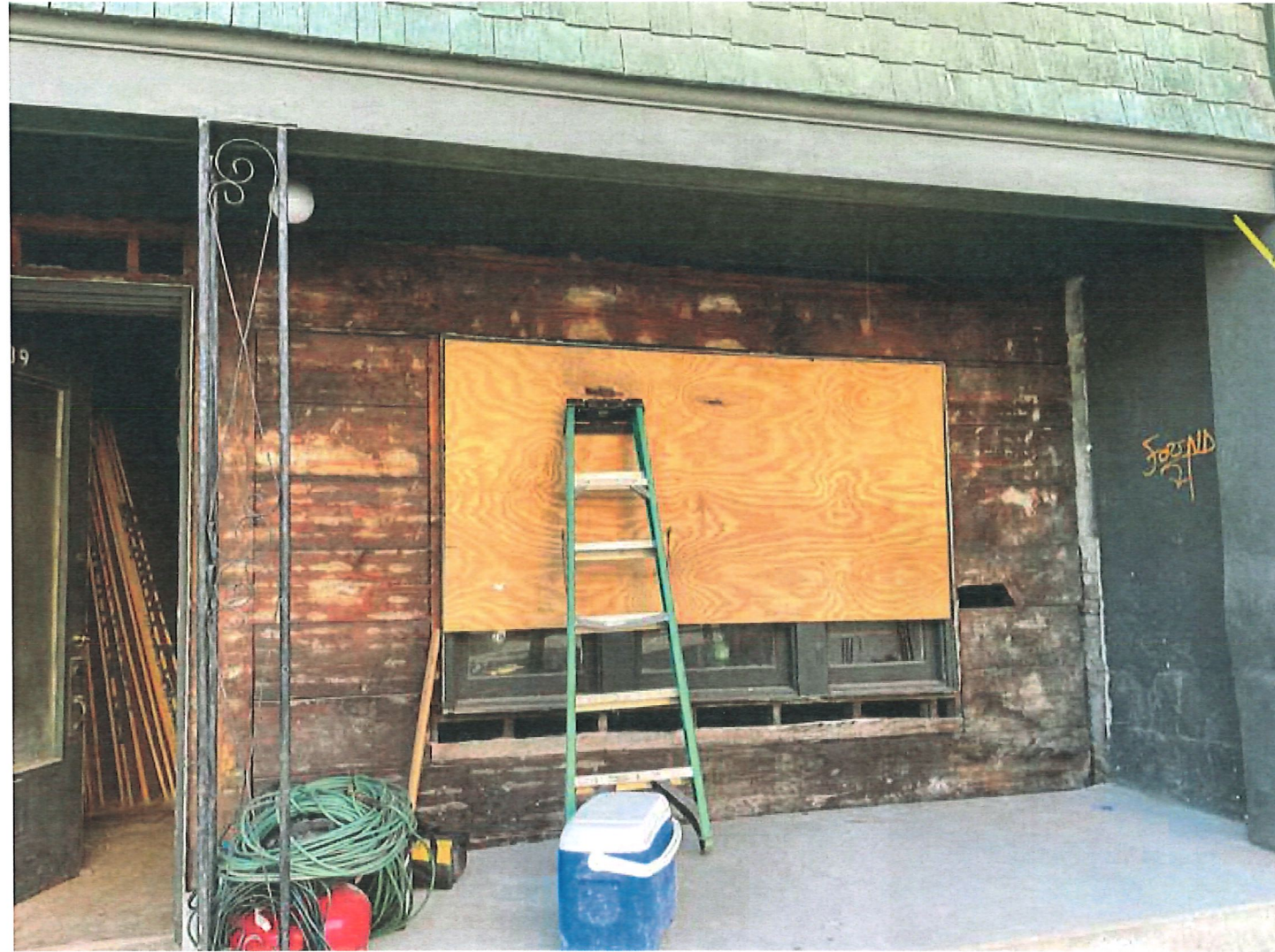
Close-up View of Recessed Wall
