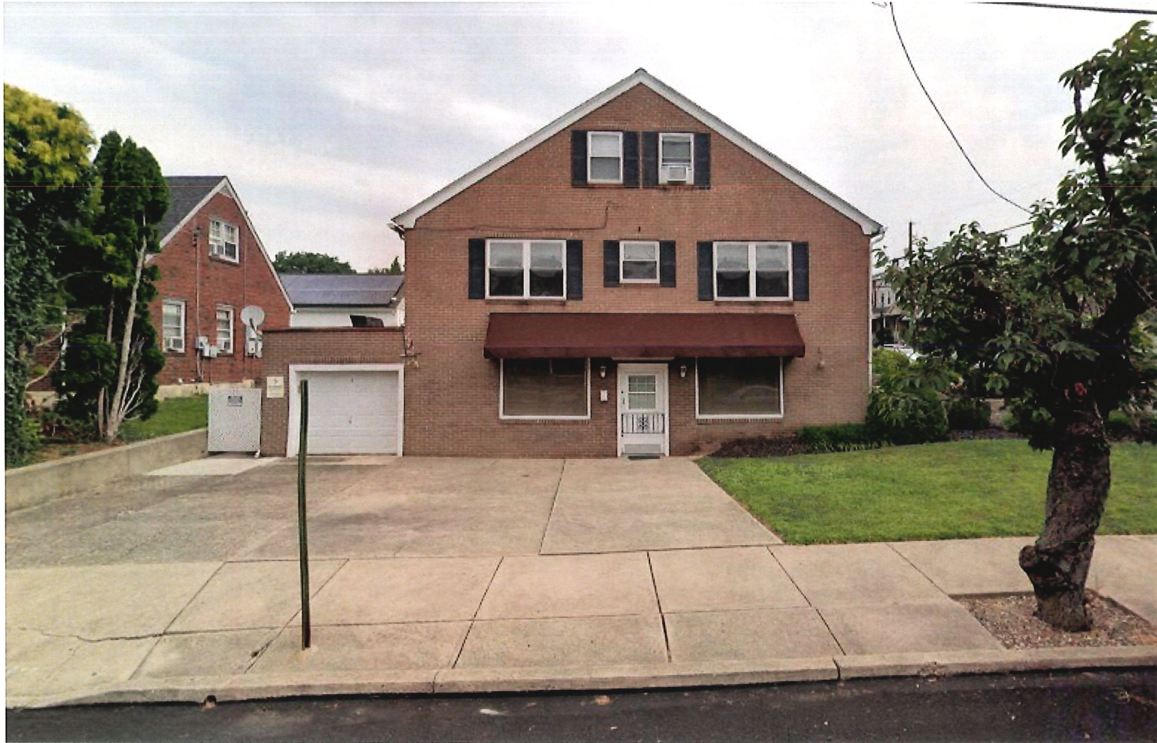
802 Spring St Existing Photos
