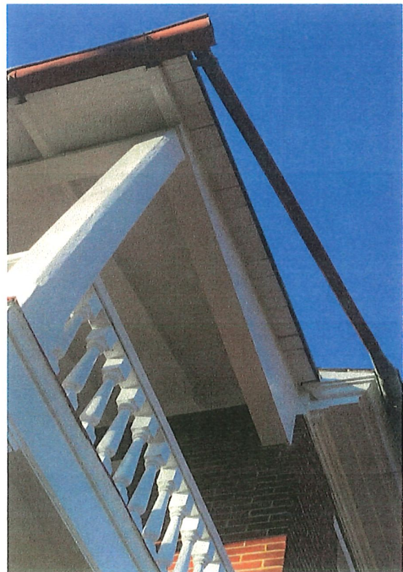
228 - Roofing, gutter, & downspout
