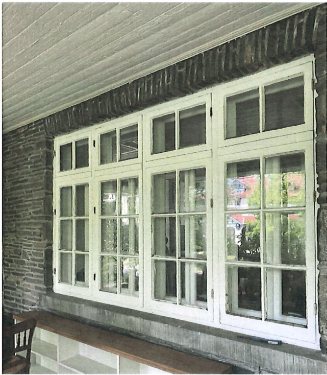
FRONT PORCH WINDOWS (NORTH FACADE)
