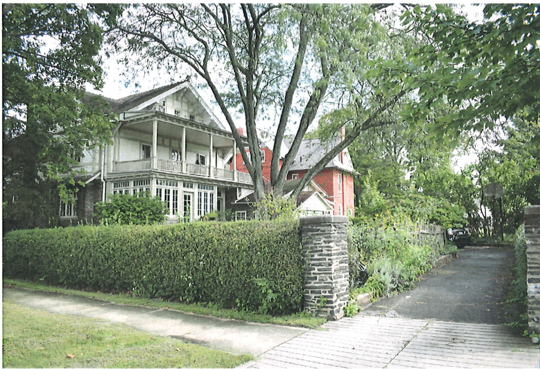
SOUTHWEST CORNER/SOUTH FACADE (LOOKING NORTHEAST)
