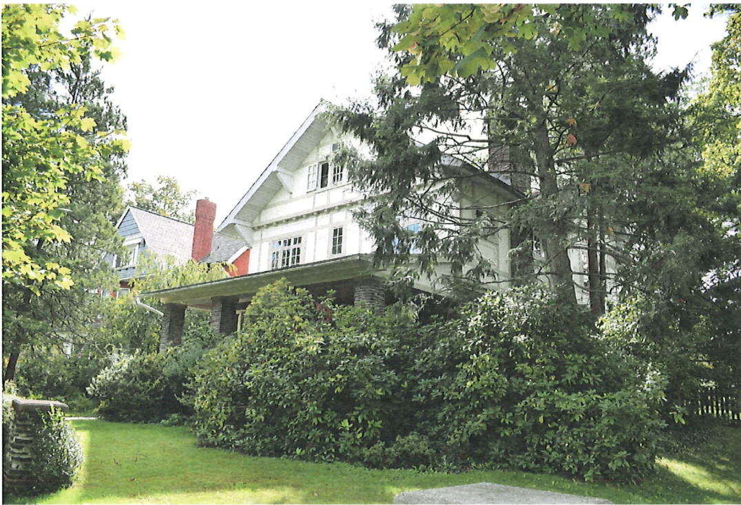
FRONT FACADE AT NORTHWEST CORNER (LOOKING SOUTHEAST)
