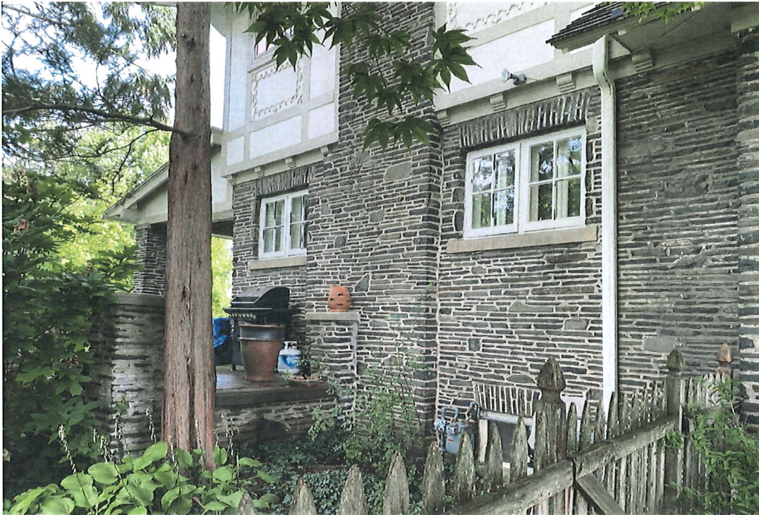
LIVING ROOM WINDOWS (WEST FACADE); TO BE LOWERED
