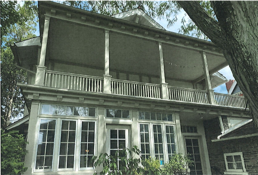
SUNROOM WINDOWS, SOUTH FACADE
