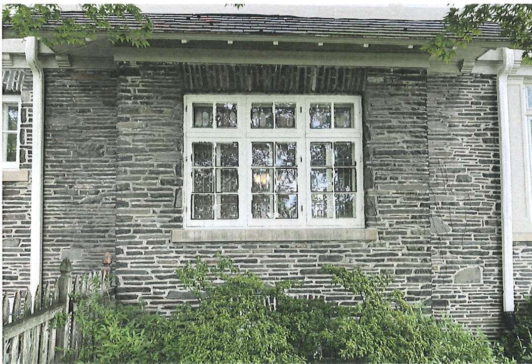
DINING ROOM WINDOWS (WEST FACADE)
