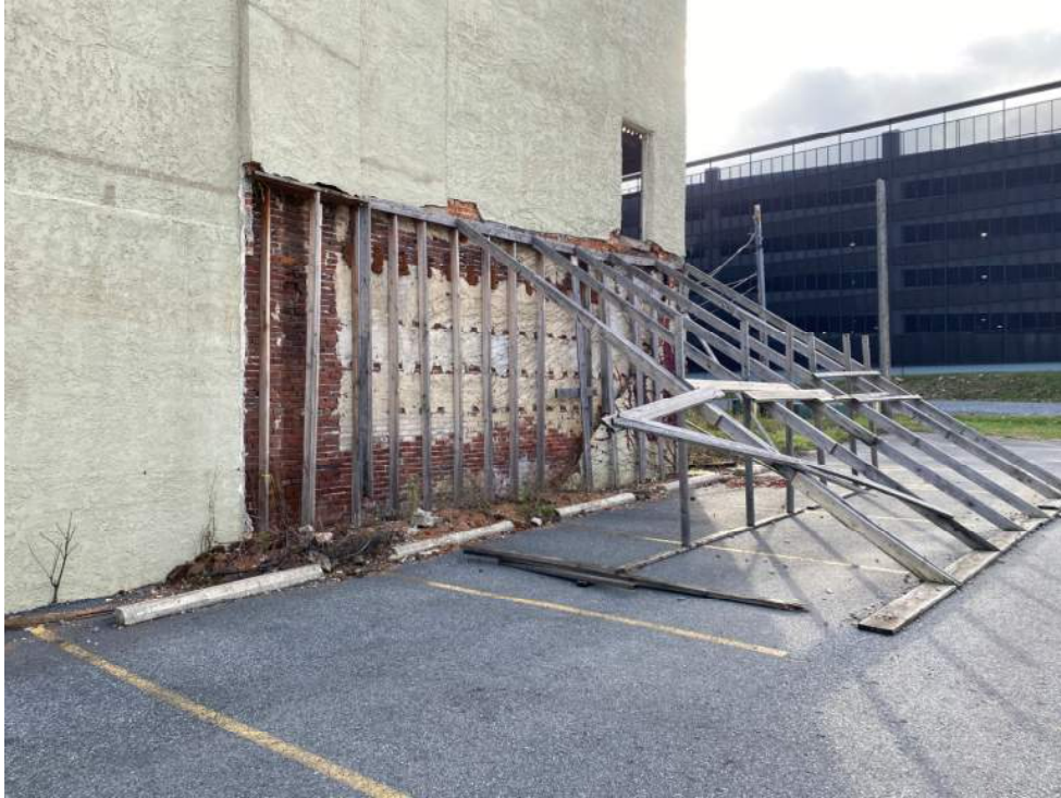
Photo 7 – Shoring on west wall.
