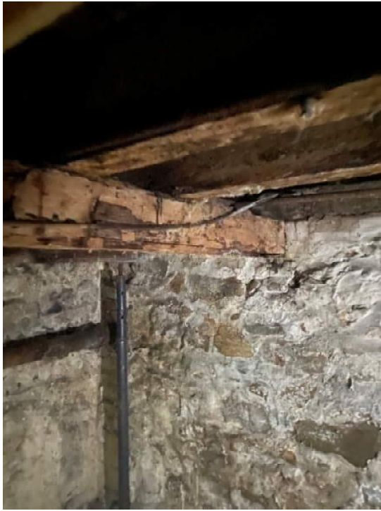
Photos 1 and 2 – Deteriorated floor framing.
