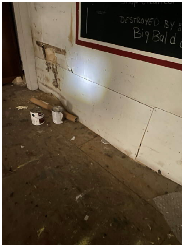
Photo 8 – Interior of west wall.
