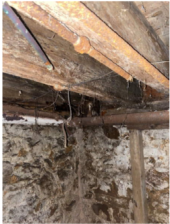
Photos 1 and 2 – Deteriorated floor framing.
