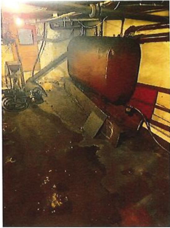
Oil Tank and Concrete Floor
