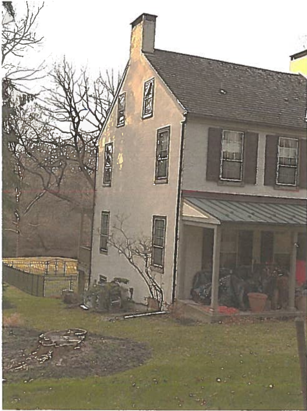
South side of house, front corner
