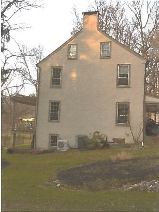
South façade of house
