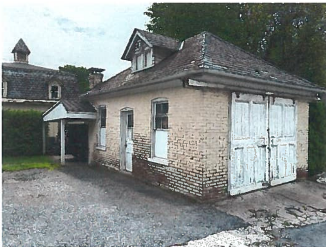
Northwest corner of garage
