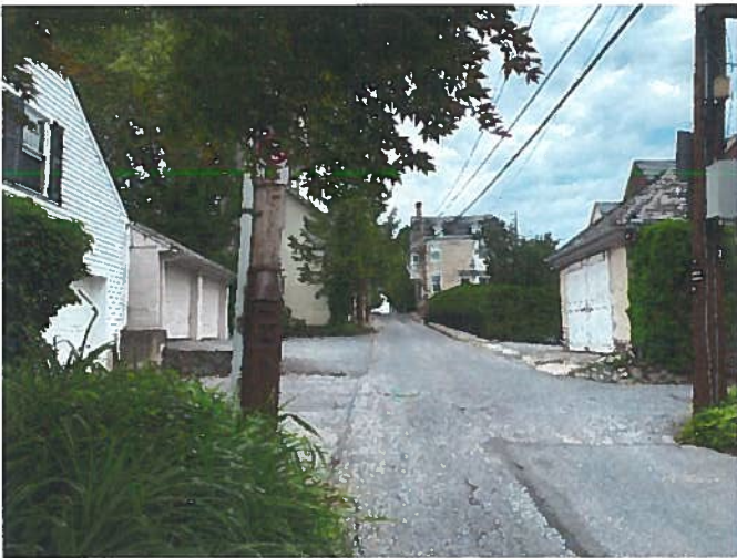
View North on Long St. from Milton St. (garage on right)
