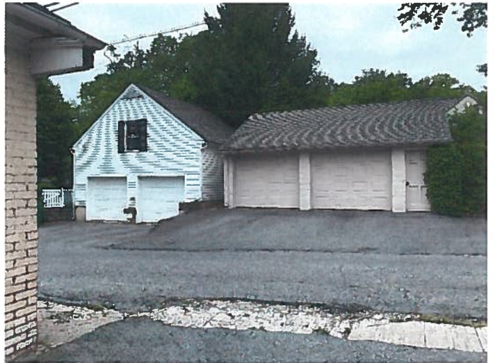
Garages behind 452 & 456 N. New St.
