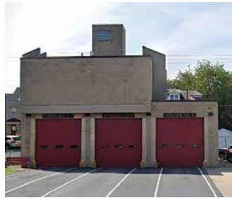
Memorial Fire Station.
