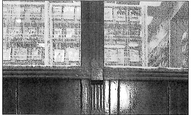
The fluted wood structural supports separate large display windows and defines the sections of the apron below.
