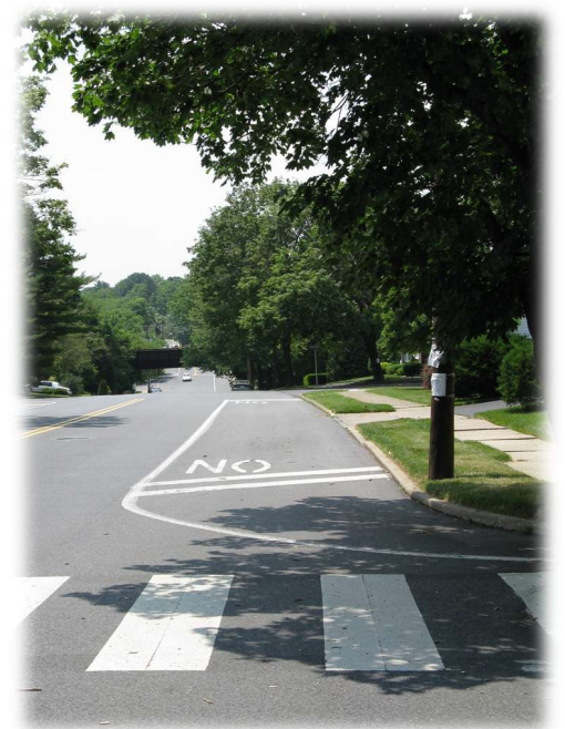
Edge line striping on Eaton Avenue
