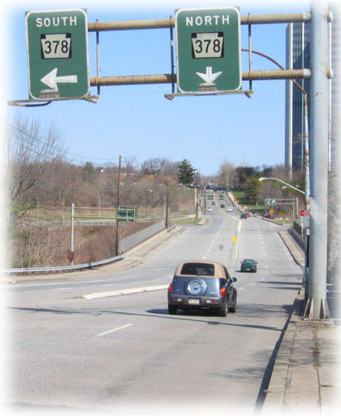
The 8th Avenue interchange of Route 378
