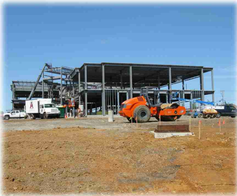
New office construction at LVIP VII
