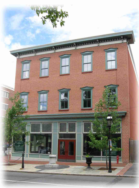
New construction has replaced a fire-ravaged structure at Broad and Main Street
