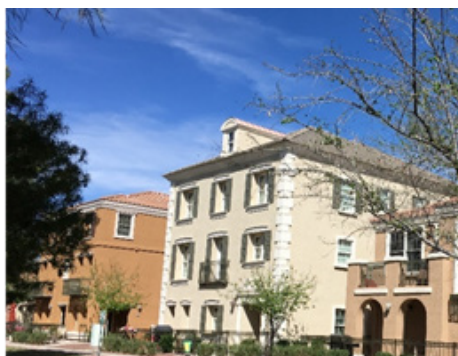
New Construction 4-Story Condo Building
