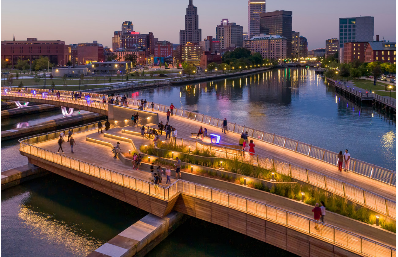
FIGURE 39. PROVIDENCE PEDESTRIAN BRIDGE
