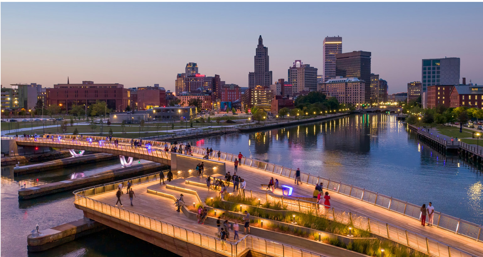
PROVIDENCE RIVER PEDESTRIAN BRIDGE (IMAGE SOURCE: WWW.BUROHAPPOLD.COM)
