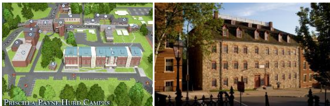
Figure 18: Moravian College’s Priscilla Payne Hurd Campus occupies a portion of the North Historic District in downtown Bethlehem, including several historic buildings such as the Brethren’s House (right), built in 1748.
