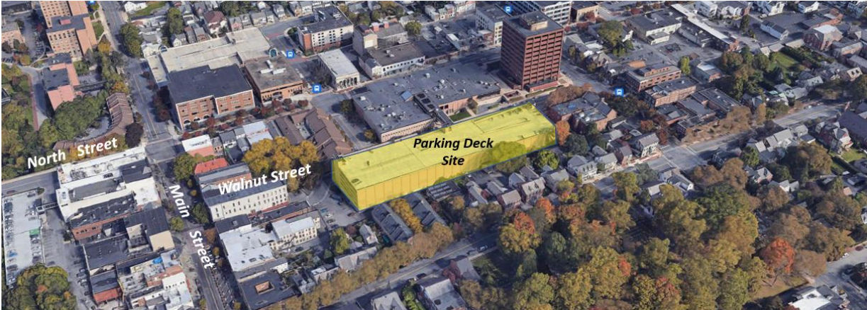
Figure 1: View of Walnut Street parking structure site looking north.
