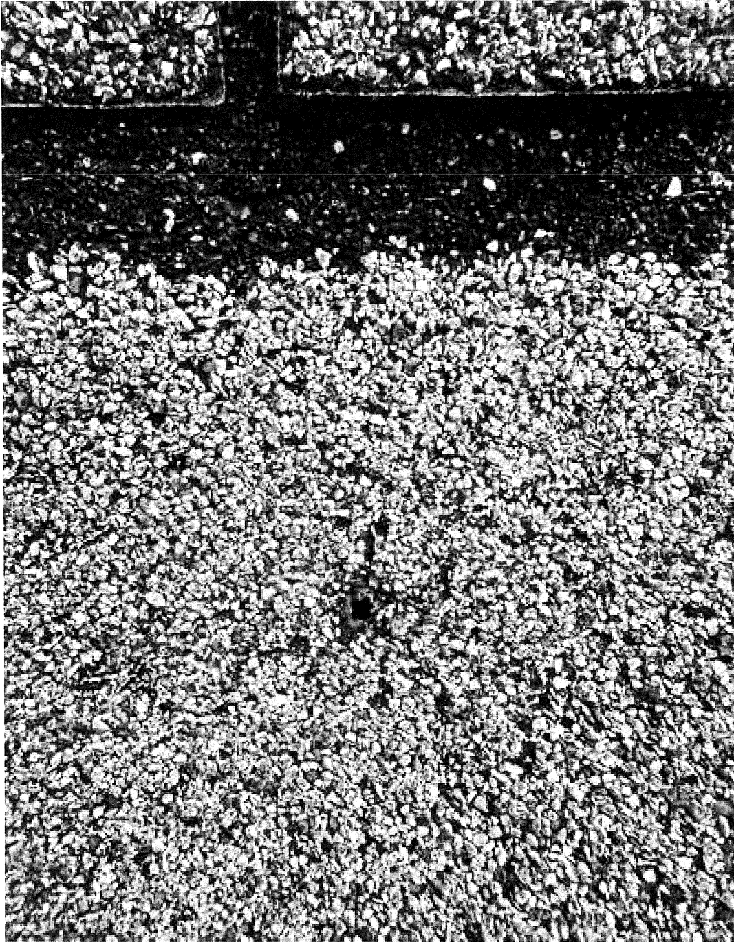
• Nail hole, cause by nails backing out
